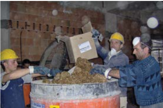
Workers adding fibers to overlay concrete mixture
