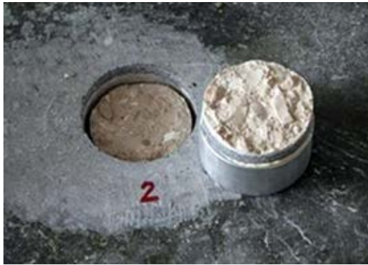
Core of floor showing bonding of overlay to existing concrete
