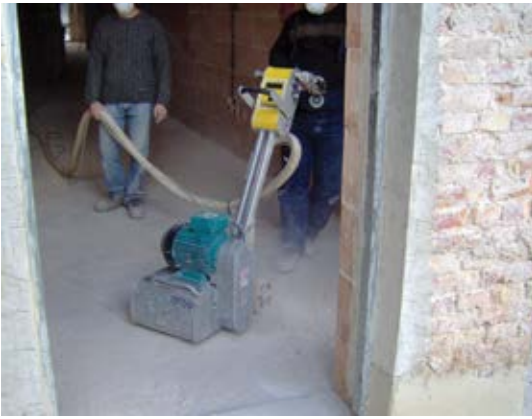
Scarifying existing concrete floor to prepare surface for overlay
