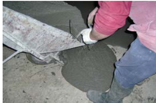
Workers placing overlay mixture
