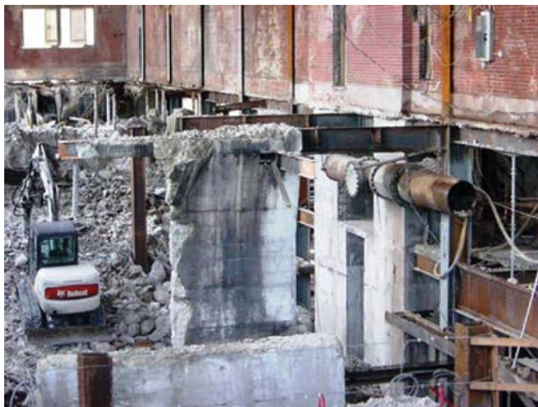
View of basement demolition
