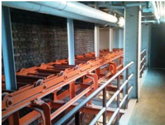
Restored conveyor system
