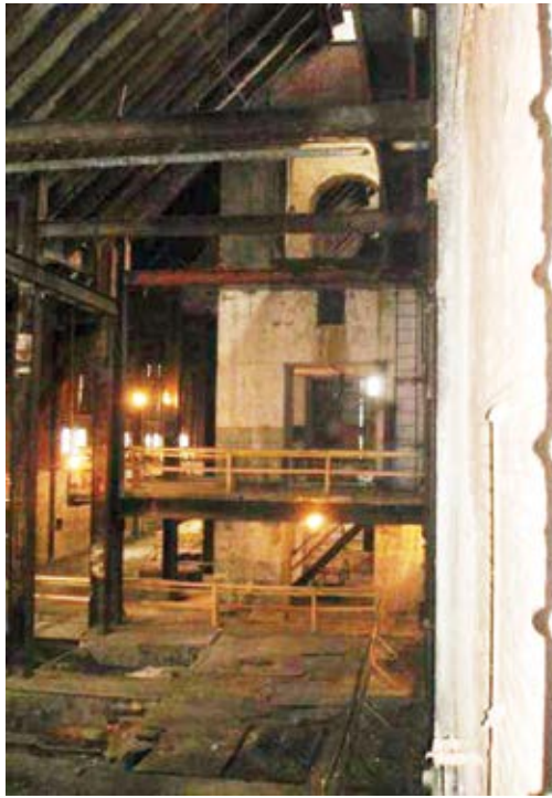
Interior after selective demolition
