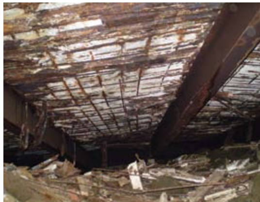
The underside of the existing ramp prior to repair
