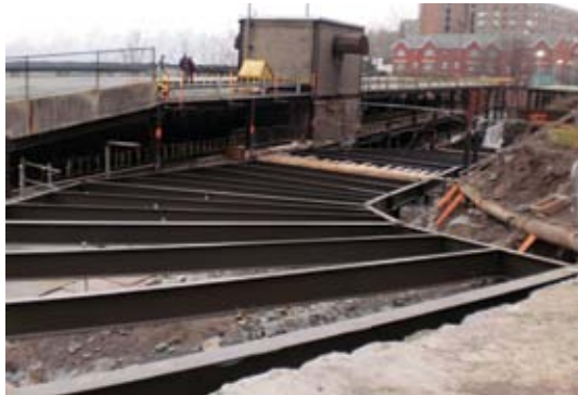
Looking down the ramp after new structural steel was placed
