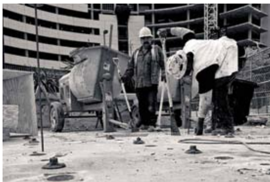
Workers placing concrete through holes in deck
