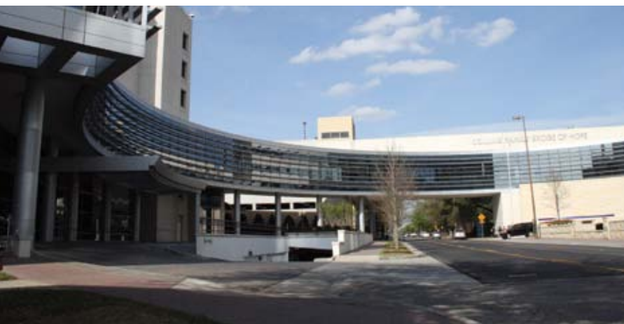
The completed Bridge of Hope
