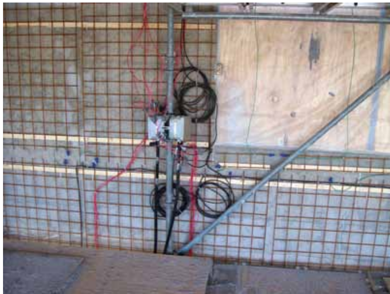
Setup for realkalization without absorbent media cover
