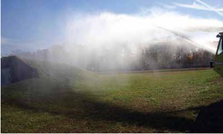
After system installation, ECM is saturated with water for testing
