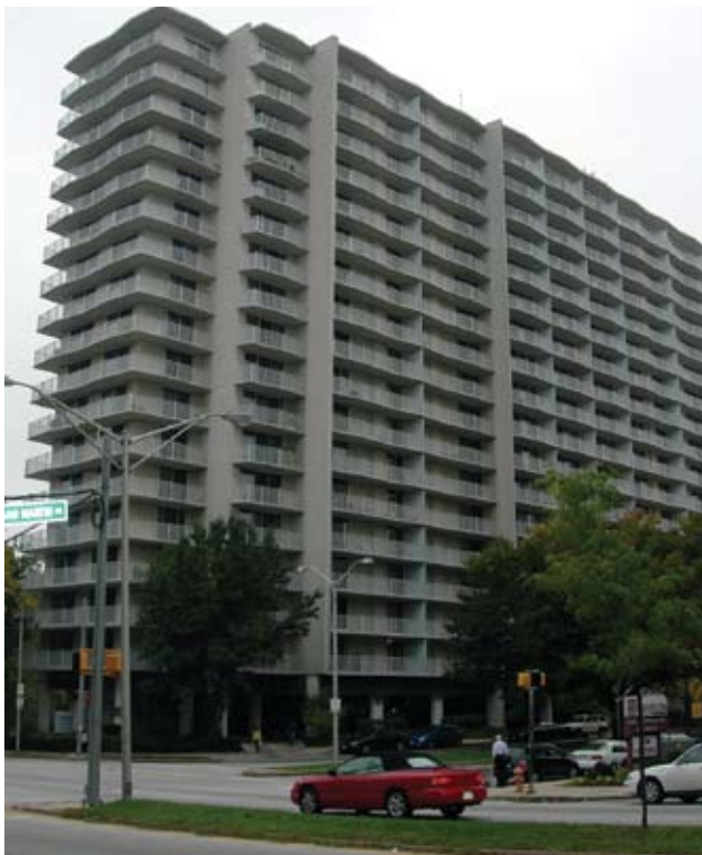
Concrete repairs, pedestrian duty coatings installations, masonry repairs, new handrail installations, and new window installations were all performed during this project
