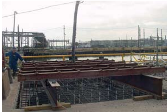
Lowering of concrete hose to place final section of dock
