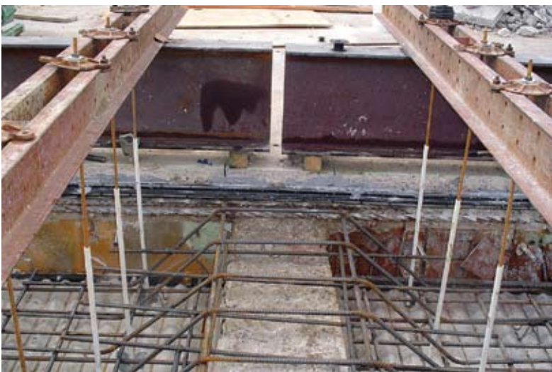
Reinforcing steel being installed; bottom layer of a double reinforced system
