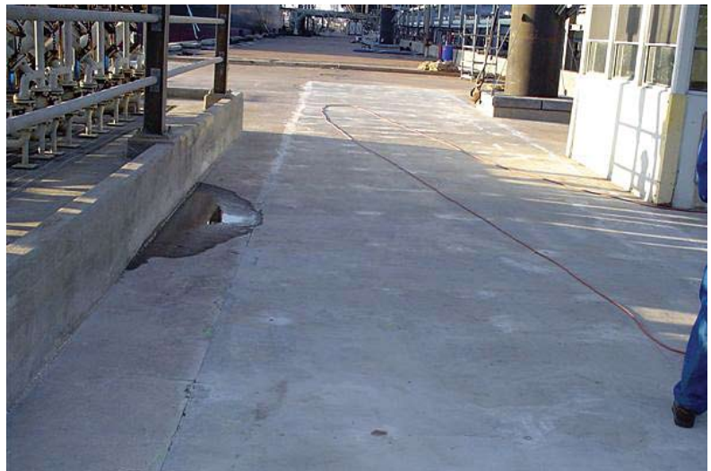
Finished shot after removing forms and filling PVC holes with grout
