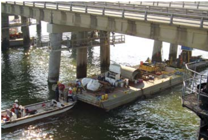
Work platforms and scaffolding under the bridge
