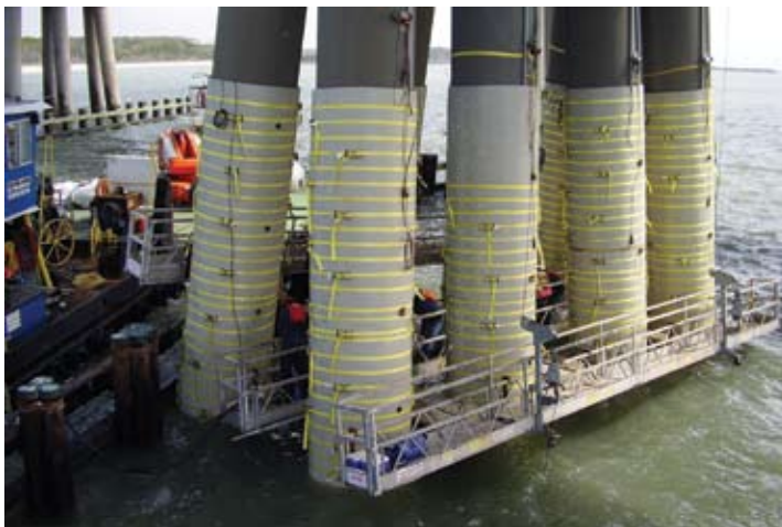
Jackets strapped into place to maintain uniform shape during grouting operations
