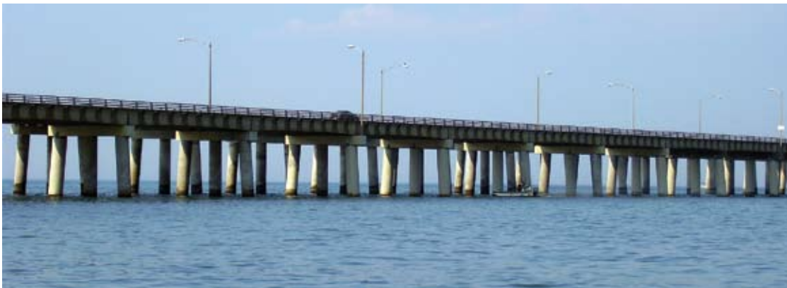
Overall view of bridge structure
