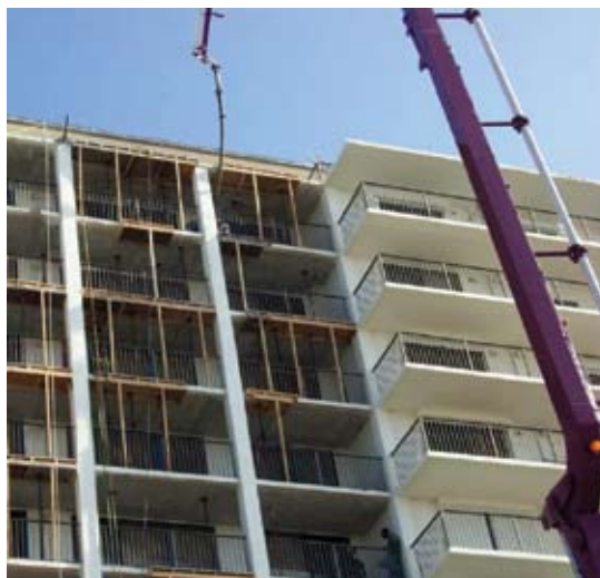
A view of the edges and balcony work
