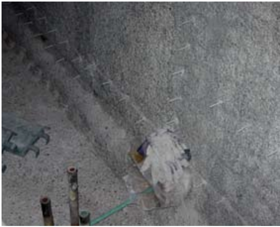
Concrete ready for epoxy injection
