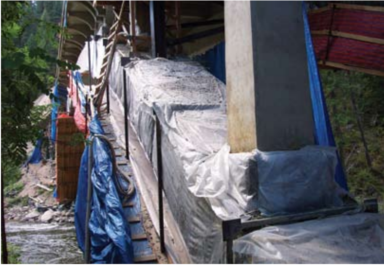
Fig. 11: ECE treatment in progress
