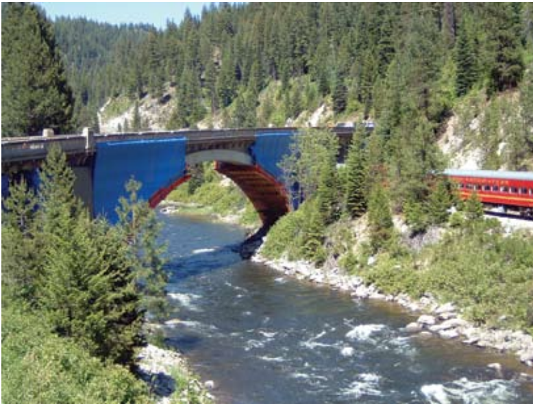
Fig. 6: Work area enclosed to protect environment
