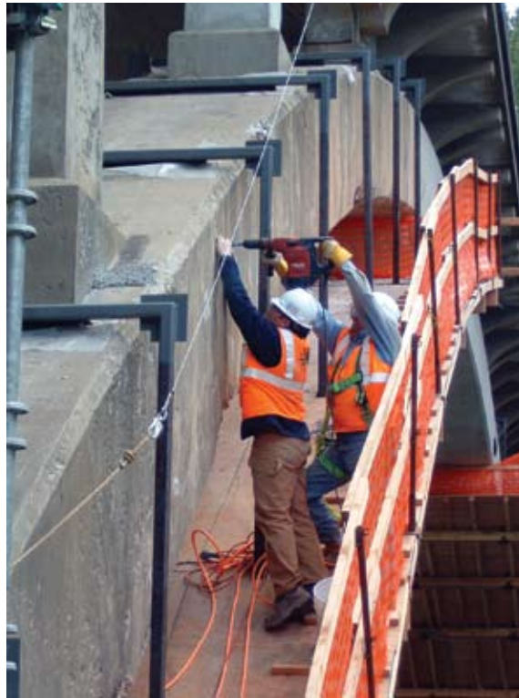
Fig. 9: Installation of reinforcing steel (cathode) connections
