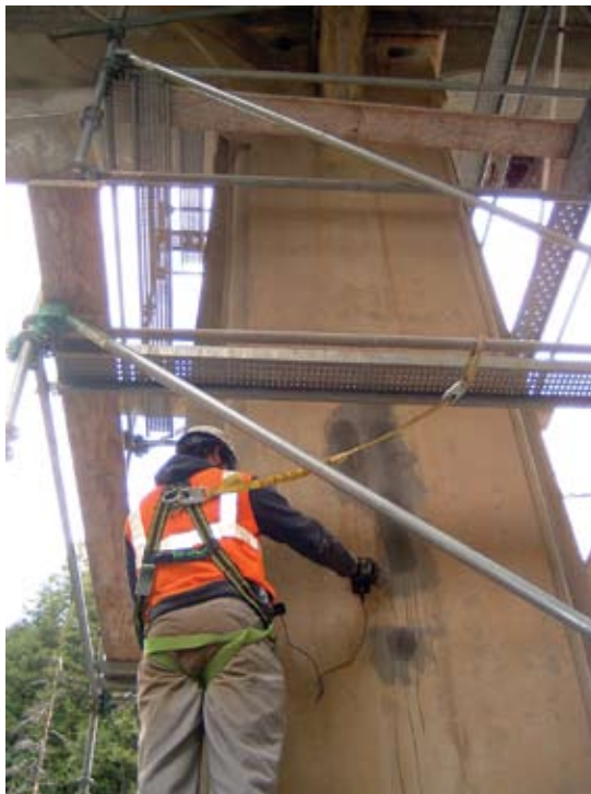
Fig. 7: Reinforcing steel cover survey before ECE installation
