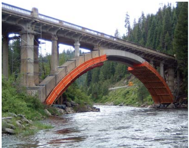
Fig. 5: Hanging platform access to the arches
