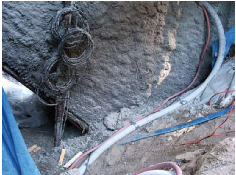
Fig. 10: Cellulose fiber installed over anode mesh
