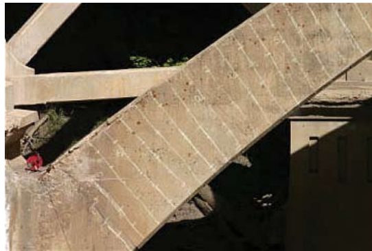
Fig. 4: Mapping grid for the corrosion potential survey
