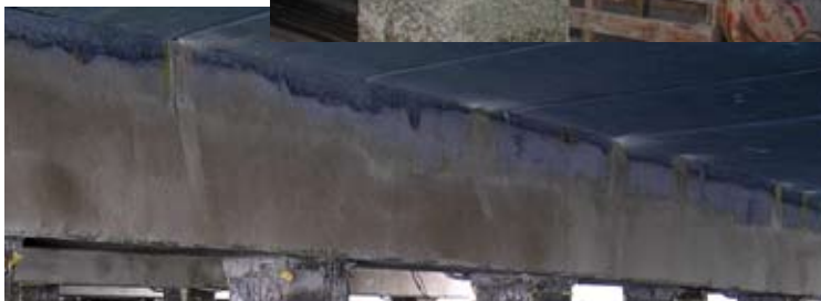
Finished pile cap repair
