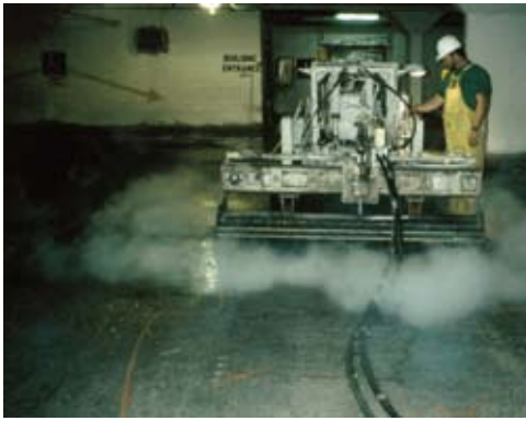
Hydrodemolition removal of deteriorated concrete
