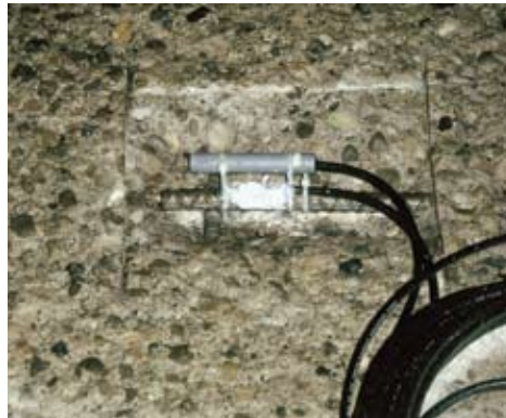
Cathodic protection reference electrode installation
