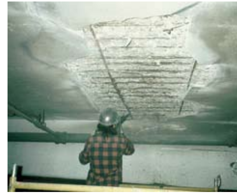
Concrete ceiling repair demolition
