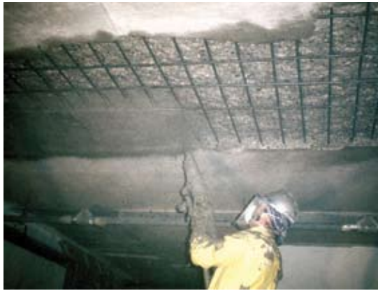
Ceiling shotcrete installation
