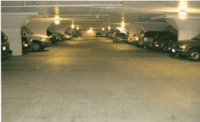
The successful repairs in April 2007
