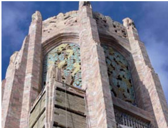
Close-up of beautiful coquina brick on Bok Tower
