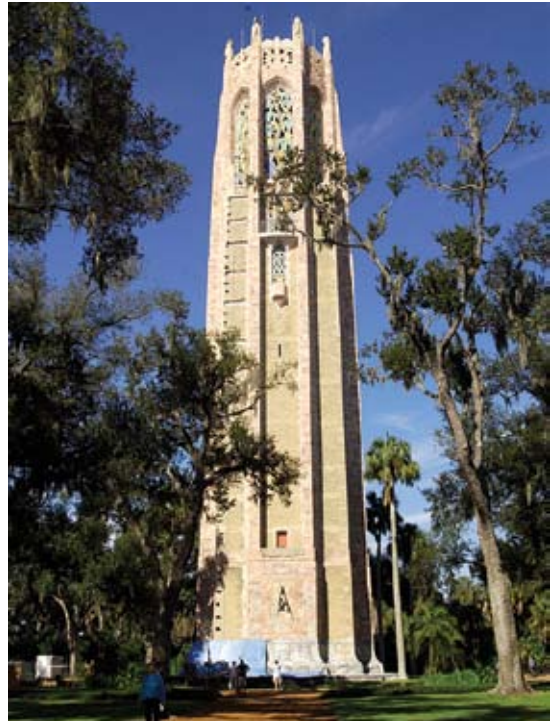
Fully repaired Bok Tower
