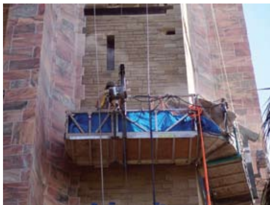
Coquina brick replacement
