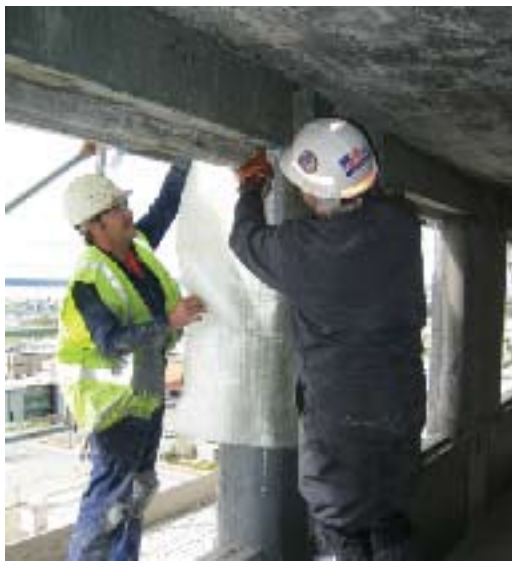
Fig. 5: Reinforcing boundary elements in shearwalls with GFRP
