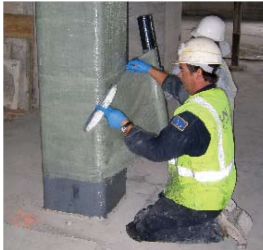
Fig. 3: Wrapping of columns with GFRP
