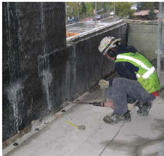
Fig. 4: Steel angles and bolts for transfer of loads from shearwalls to floors
