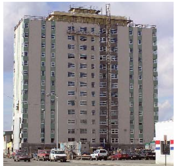
Fig. 6: The building nearly completed and painted
