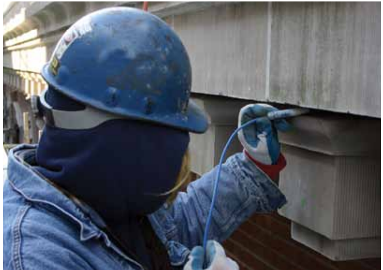
Placement of reference electrode into mortar joint above terra-cotta modillion
