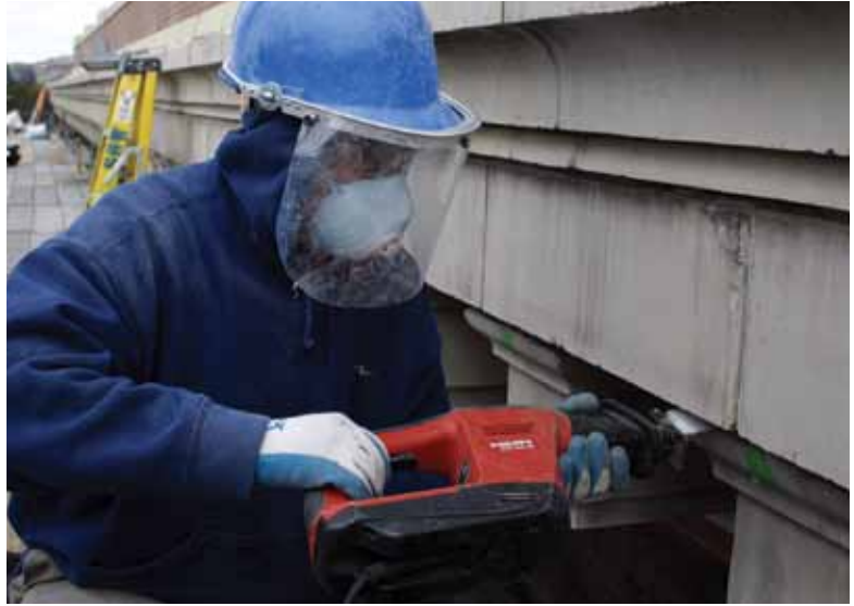
Removal of portland cement mortar joint above the terra-cotta modillions
