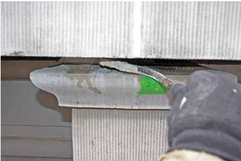
Placement of lime-based mortar after anode and reference electrode installation
