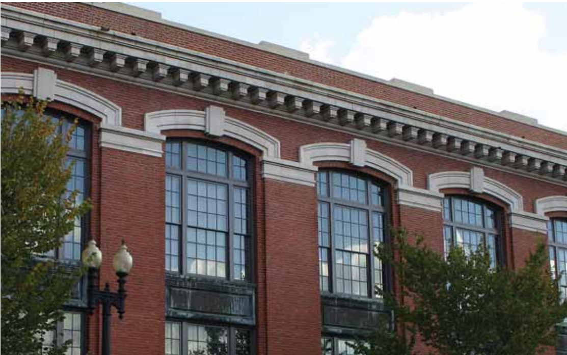
A view of the restored terra-cotta cornice
