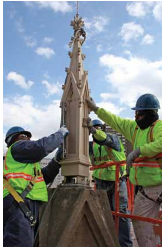
Alignment of spire in preparation for tack welding
