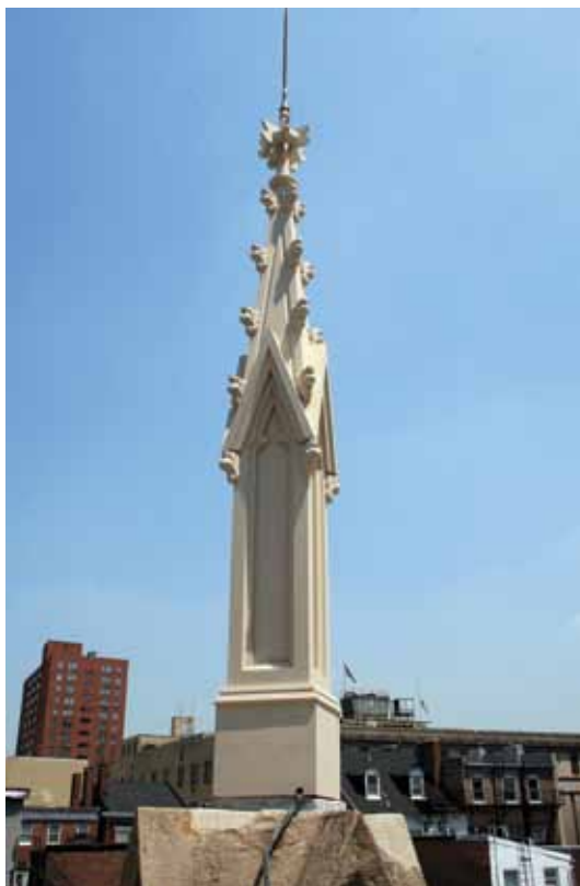
After 100 years, the original gothic element is restored
