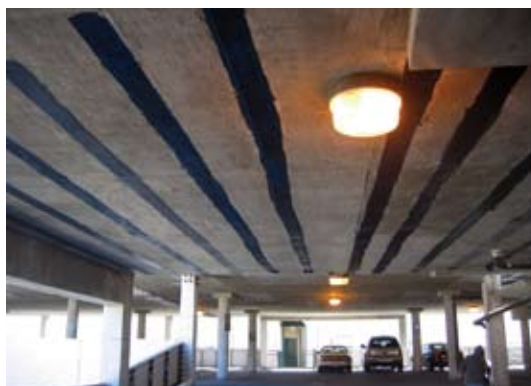
Fig. 3: Slab underside strengthened with CFRP laminates
