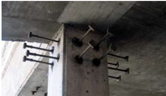
Fig. 4: Headed bars used in the construction of external shear collars
