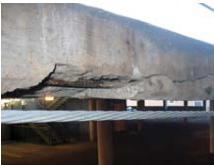
Fig. 5: Cracking on slab edge shown before and after repair
