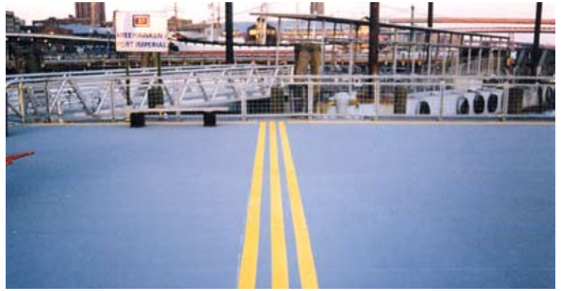
Bright yellow stripes improved safety by providing a trafficway that is visible at night
