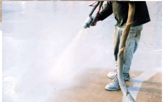
Spraying the coating
