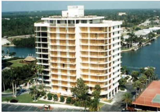
Full-scale balcony renovation project
