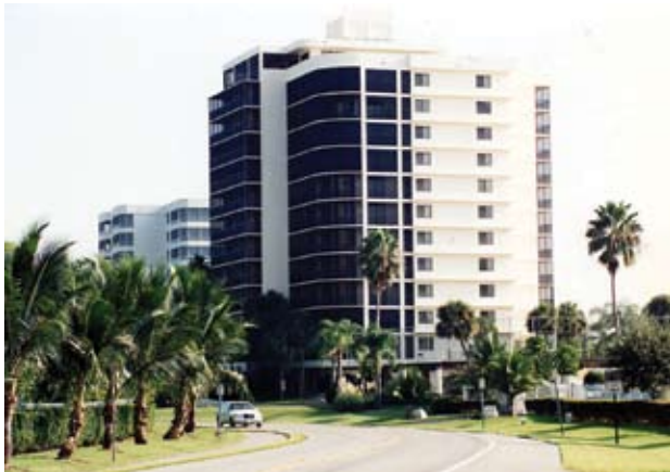
Completed balcony renovation project
