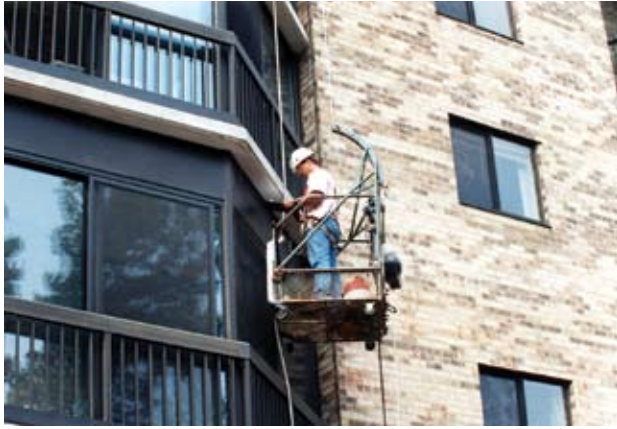
Warranty inspection using exterior swing staging. No unit access required
