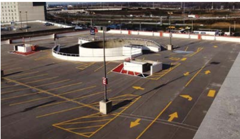
Fig. 6: Completed view of “D” garage
