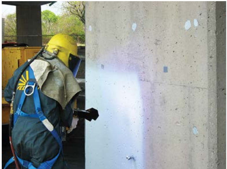
Fig. 3: Humectant-activated arc spray zinc
