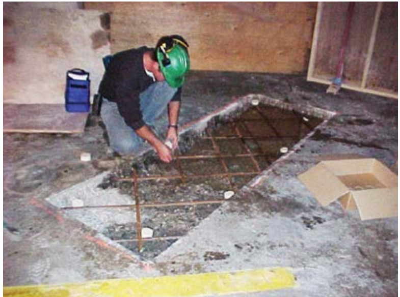
Fig. 2: Installation of galvanic anodes in repair area
