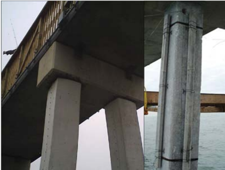
Fig. 6: Marine pile protection with self-activated distributed anodes inside FRP jacket
