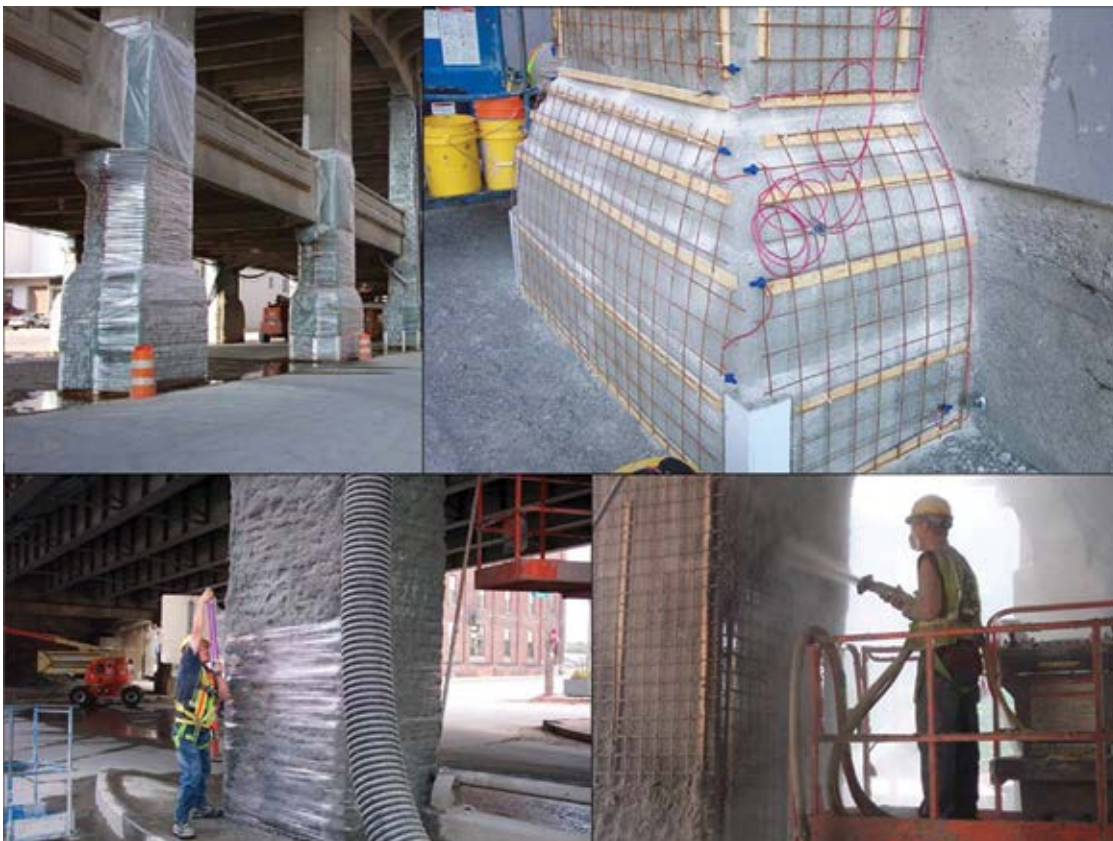
Fig. 2: Chloride extraction performed on historic viaduct
