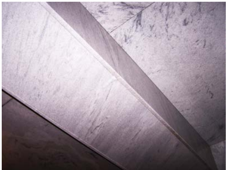
Fig. 4: Typical 18 x 18 in. (457 x 457 mm) concrete beam encasement in hallway
