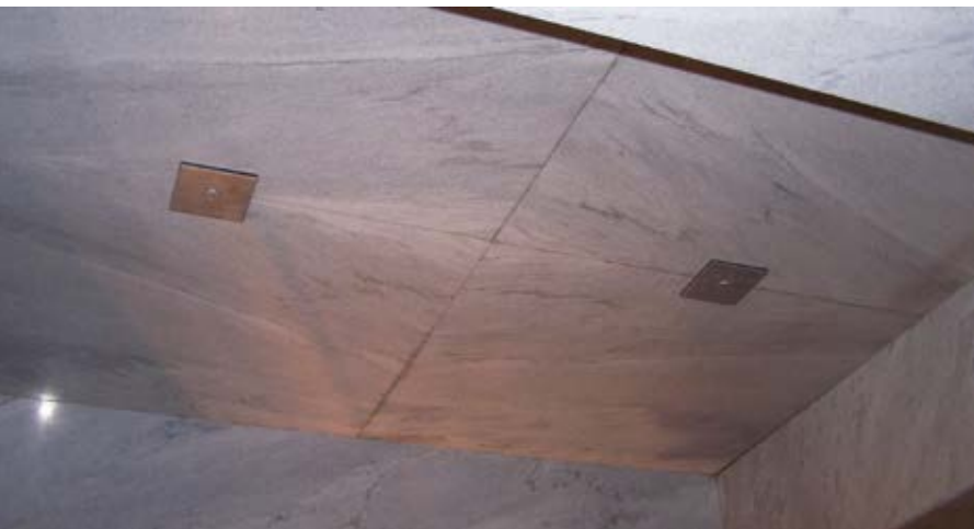
Fig. 6: Typical ceiling support assembly
