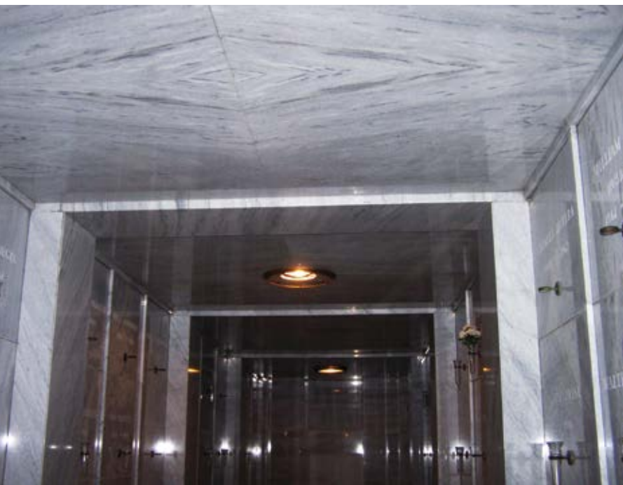
Fig. 2: Interior view with marble-clad ceiling, beams, and walls
