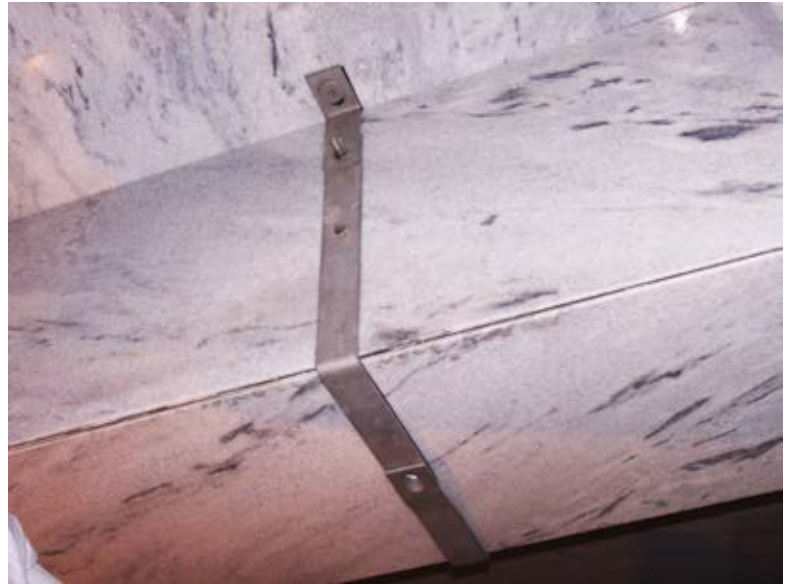
Fig. 8: Box beam encasement assembly for 18 x 18 in. (457 x 457 mm) beam
