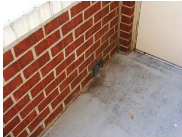
Fig. 9: Drainage outlet for existing balcony wall
