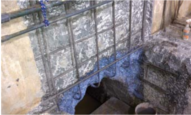
Fig. 11: Replaced reinforcing steel
