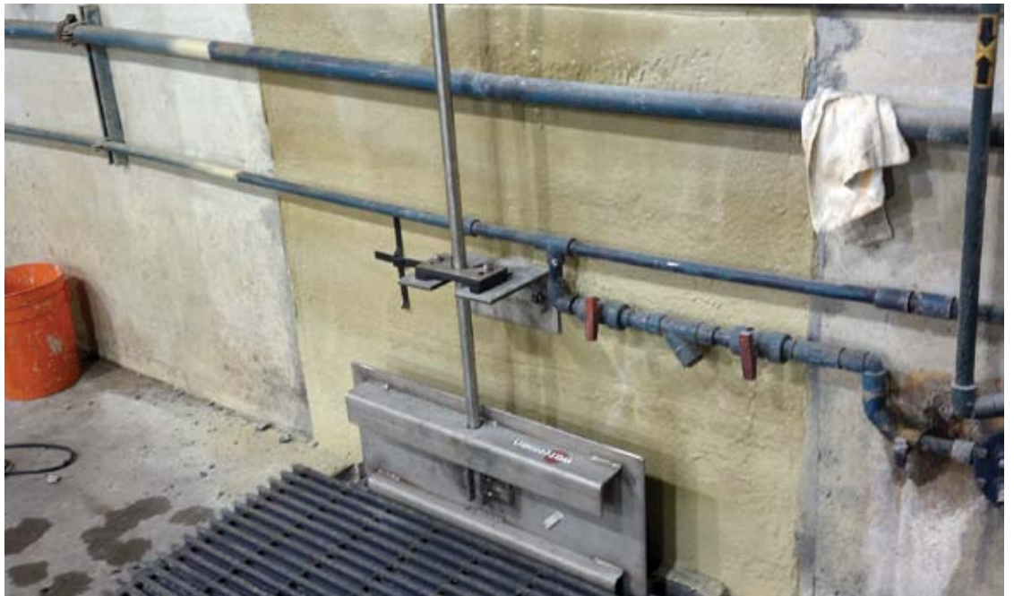
Fig. 13: Completed repaired area with the sluice gate in place
