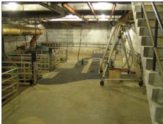
Fig. 3: Overall view of the wet well area
