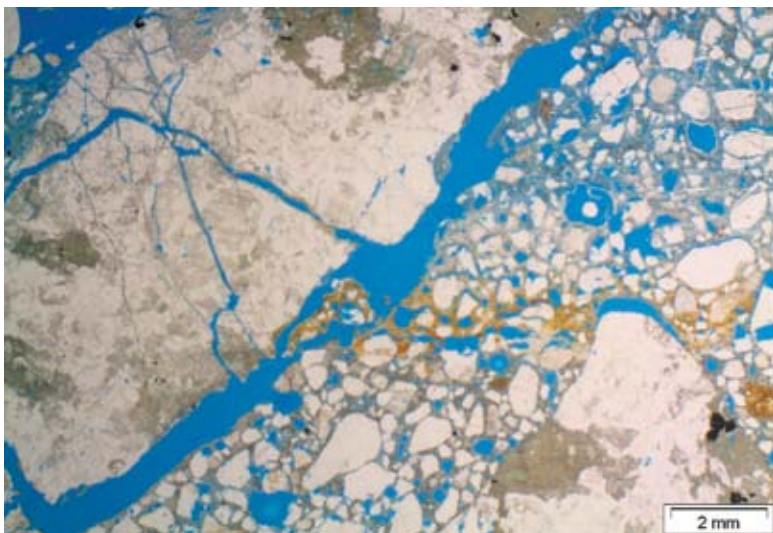
Fig. 8: Thin section of the deteriorated portion showing cracking and porous nature of concrete as indicated by the blue dye-mixed impregnated epoxy
