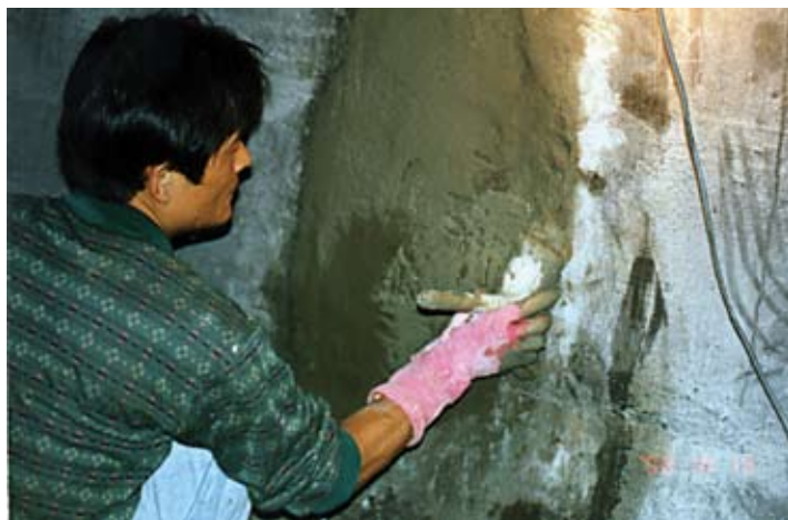
Working on concrete repairs in the Shanghai subway
