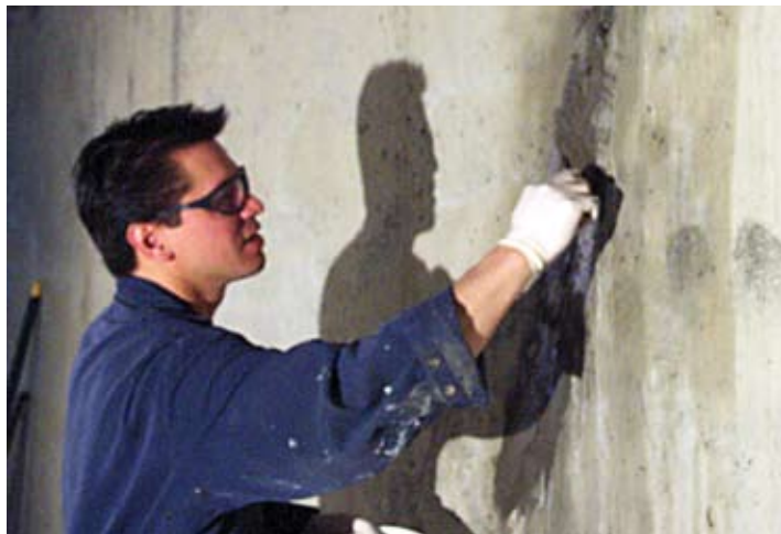
(Above and below) Crack repair using crystalline waterproofing
