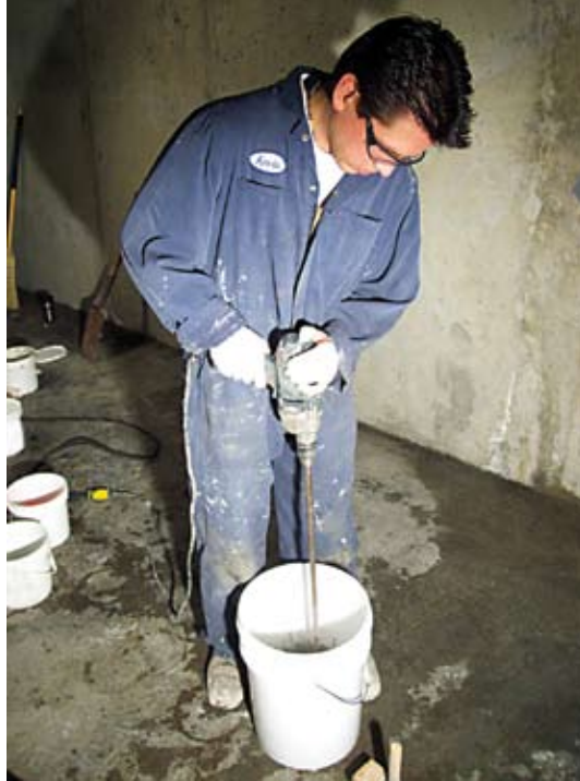
(Above and below) Crack repair using crystalline waterproofing
