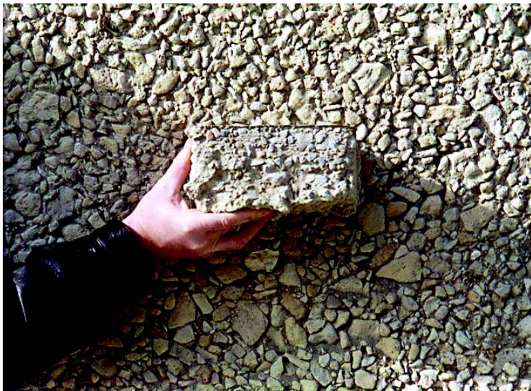
Mockup of exposed aggregate concrete
