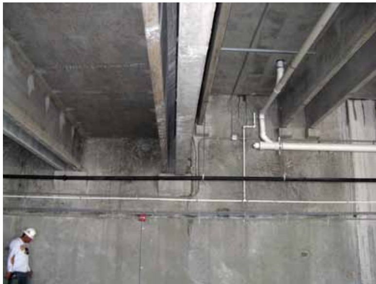
Double-tee beams before strengthening
