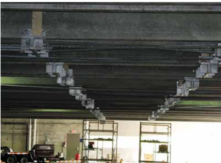
Parking garage tees after strengthening
