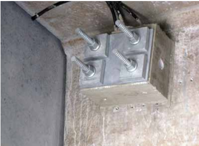
Finished anchor block
