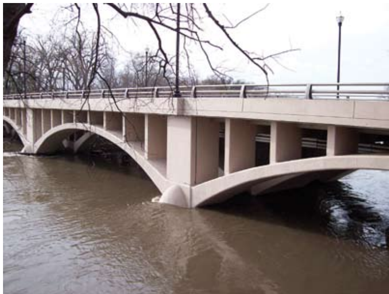
Station Street Bridge after repairs
