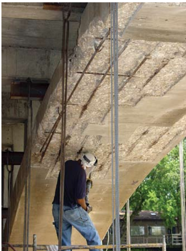
Arches being prepared for repair
