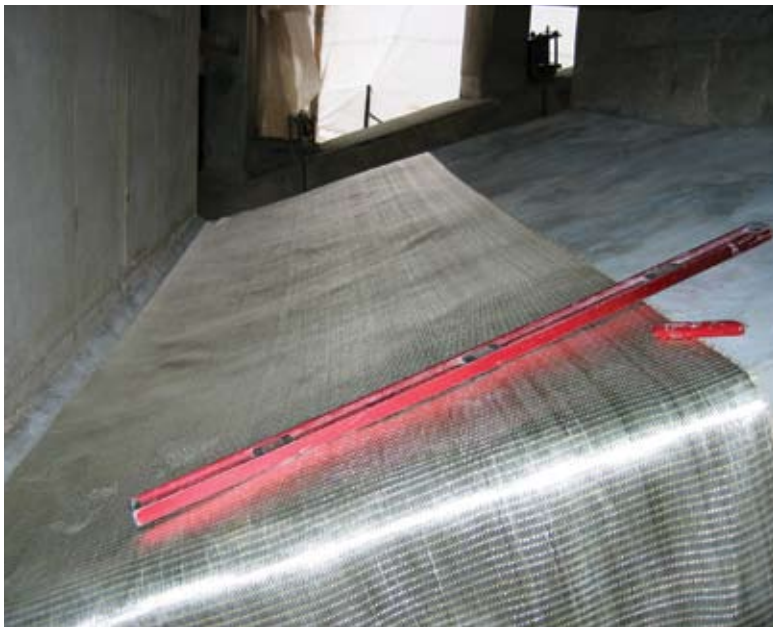
Glass fiber-reinforced polymer being measured for placement
