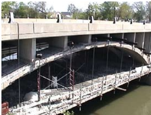
Scaffolding being erected
