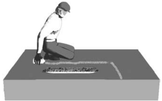
Fig. 2—Mark the perimeter of the repair area using simple geometric shapes and minimizing re-entrant corners.
