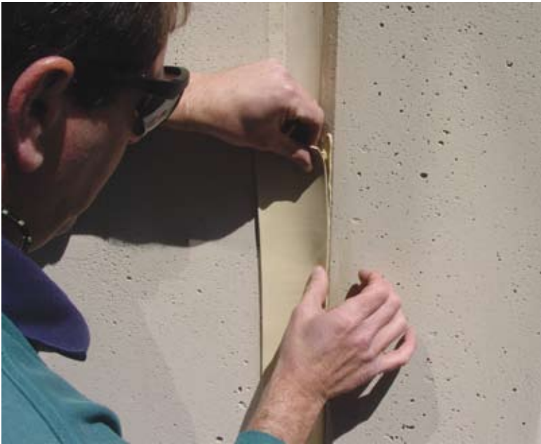
Fig. 3: Repair joint installation
