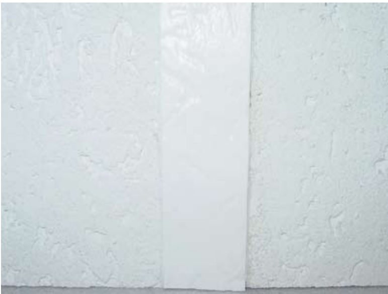
Fig. 4: EIFS joint repaired using textured pre-cured silicone sealant
