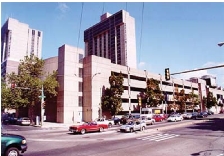
Fig 1: Exterior view of garage looking northwest
