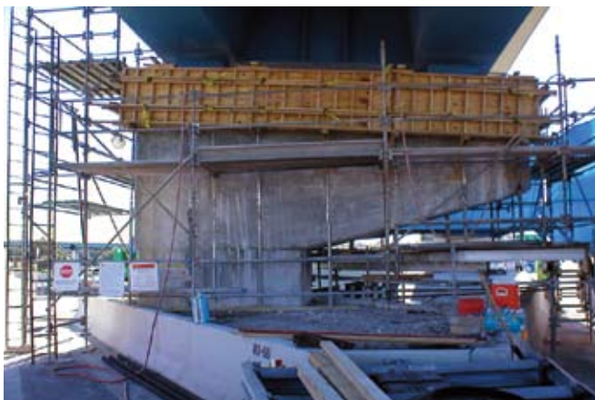
Fig. 5: Pier Two formwork for enlarged concrete pier cap section
