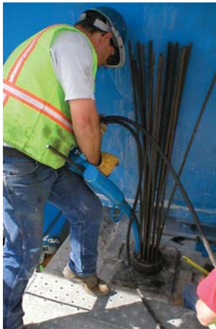
Fig. 9: Positioning of jack prior to stressing of post-tensioning tendon
