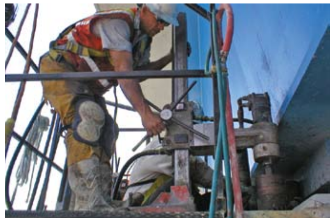
Fig. 7: Coring operation for vertical post-tensioning at Pier Two
