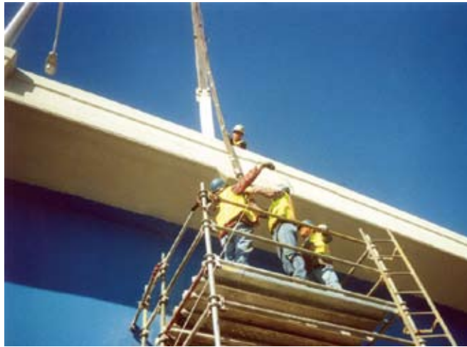
Fig. 8: Using crane to lower the post-tensioned assembly into the core hole
