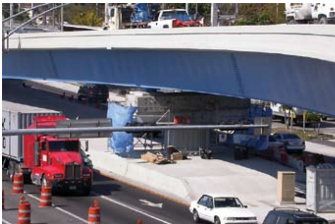
Fig. 1: Looking at Pier Three from scaffolding at Pier Two
