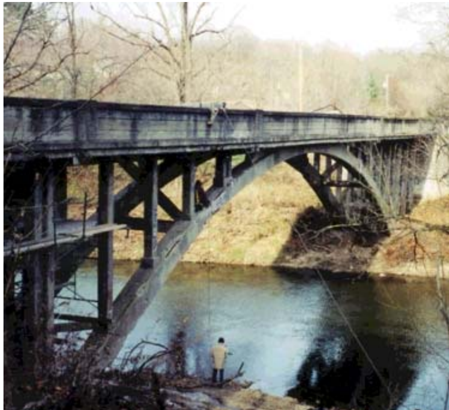
Fig. 6: Case History 3 bridge
