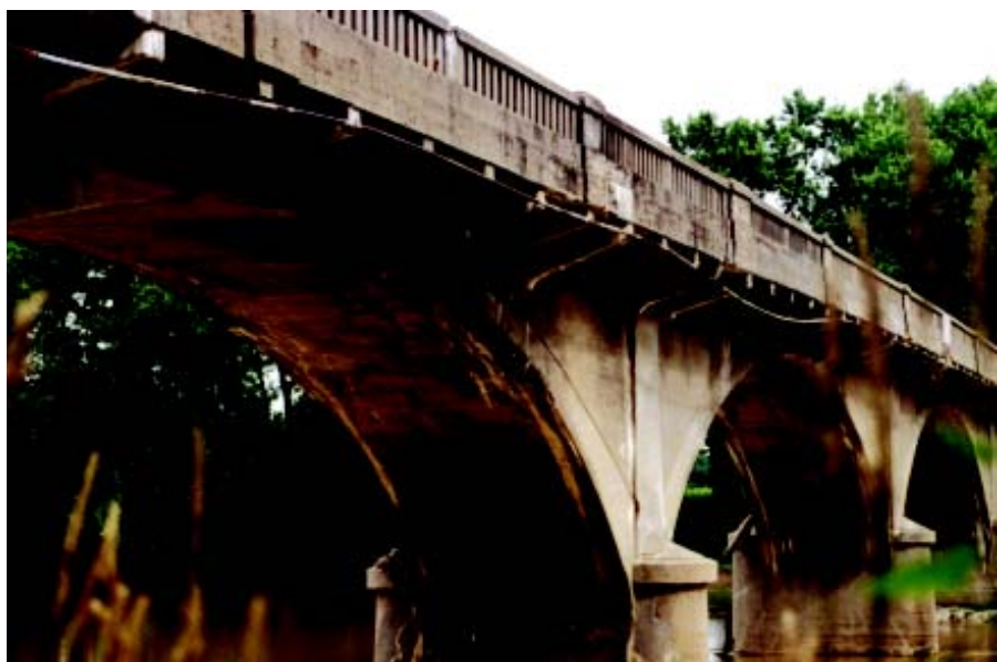
Fig. 4: Case History 2 bridge
