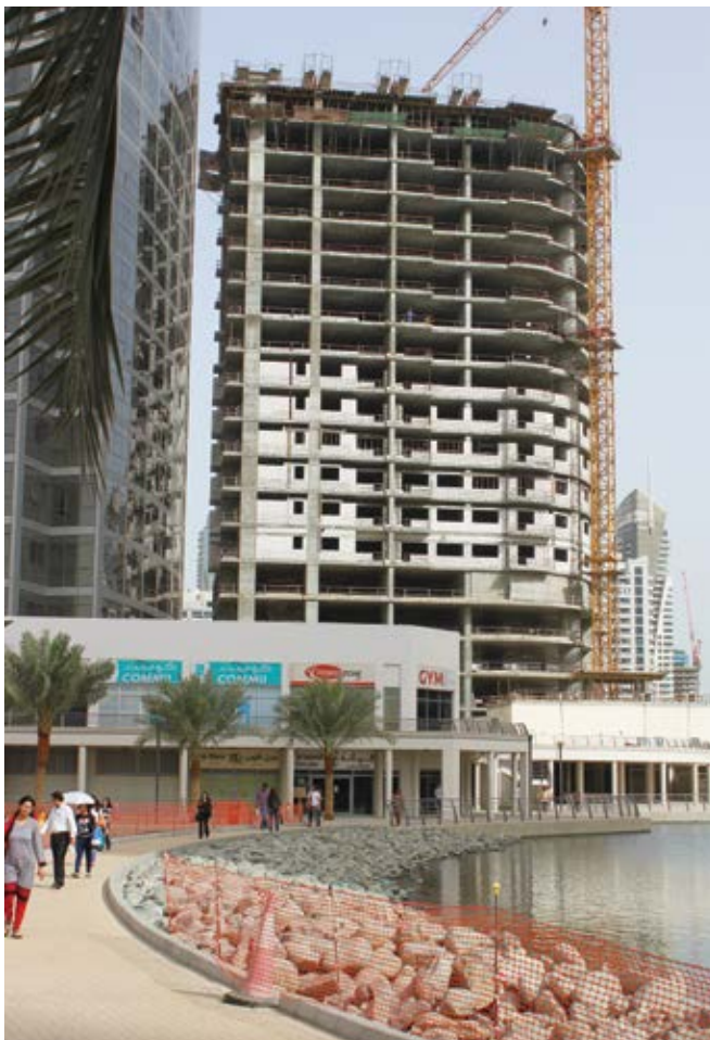
Fig. 1: The tower under construction while the water infiltration issues were occurring
