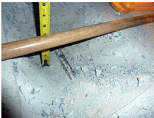
Fig. 5: Investigative test pit near column
