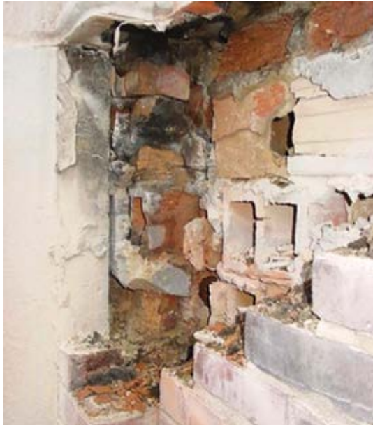
Fig. 3: Materials of different behavioral properties, including cast stone, clay brick, sand lime brick, terra-cotta tile, and polyurethane joint sealants. Previous leakage through joint sealants has caused deterioration of the brick
