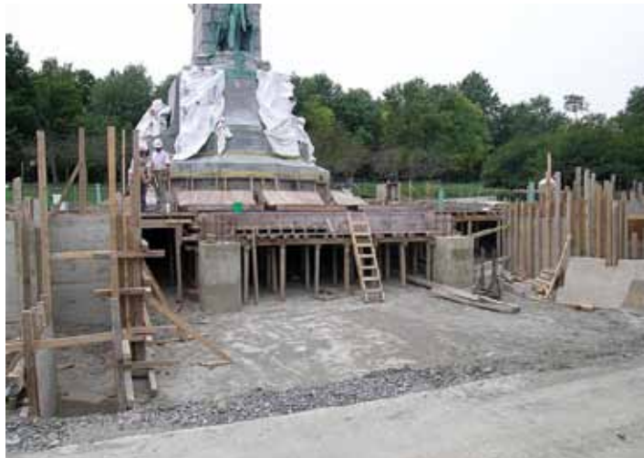
Detail of cofferdam, spring 2006 Photo courtesy of the city of Montréal
