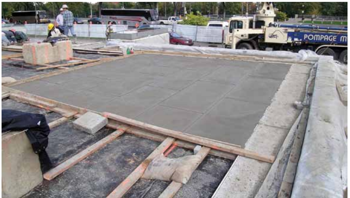
Hand crafted joints in the terrace Photo courtesy of the city of Montréal
