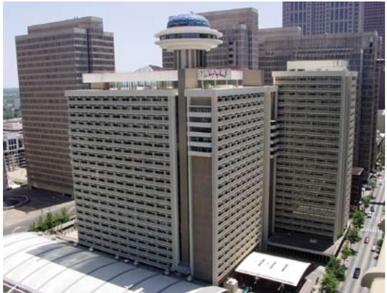
Hotel after repairs are complete
