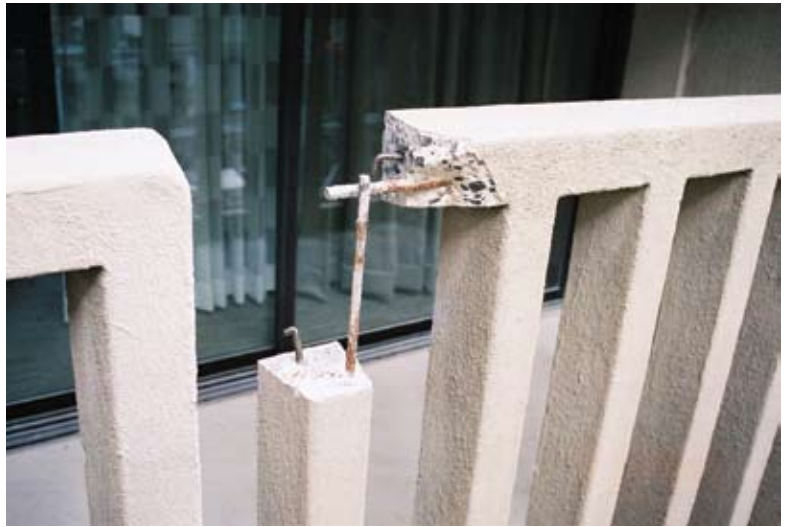
Balcony railing being prepped for repair
