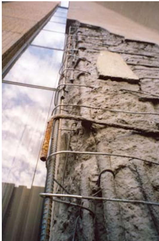
Chipped-out repair area
