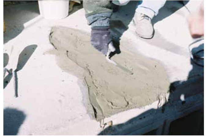
Repair mortar being applied
