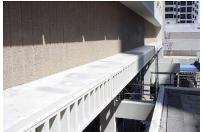
After repair and coating
