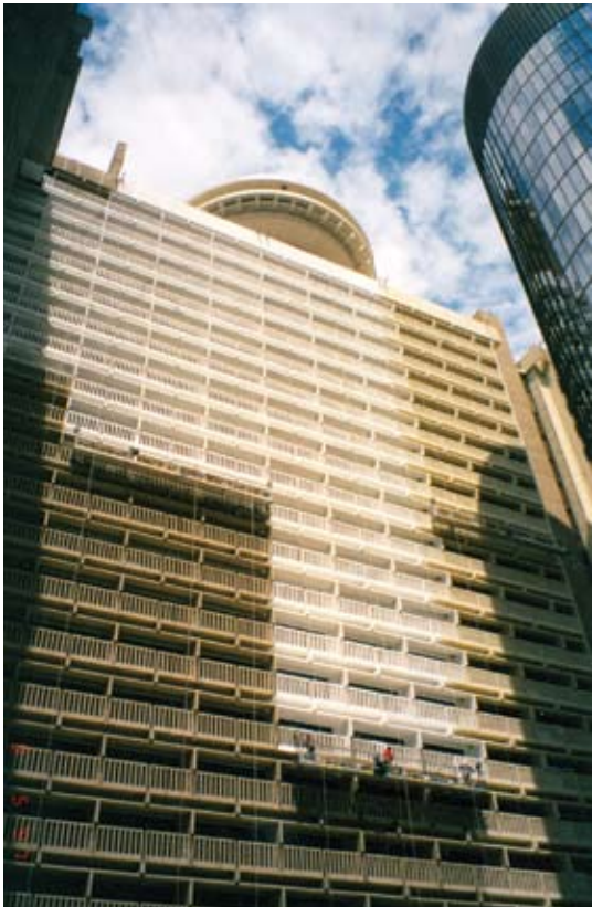
Balconies being repaired
