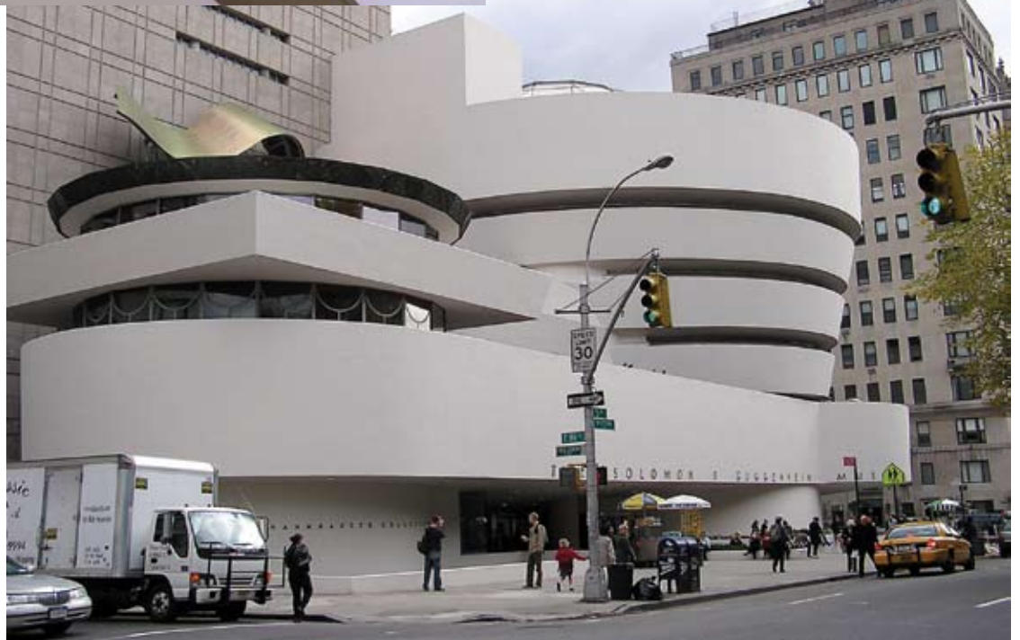
Frank Lloyd Wright's Guggenheim Museum, built in 1959 in New York, was coated with a highly breathable acrylic elastomer in 2004
