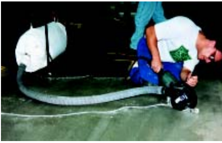
Crack chasing with dustless equipment.
