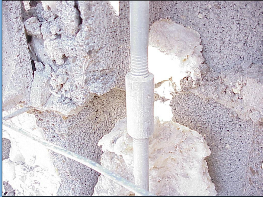
Coupler installation
