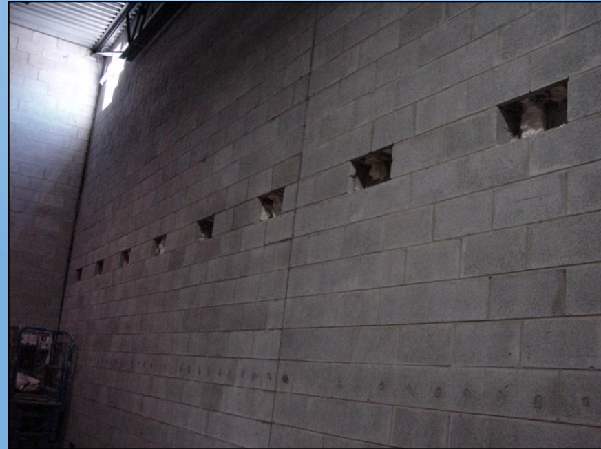
CMU cells removed for coupler
