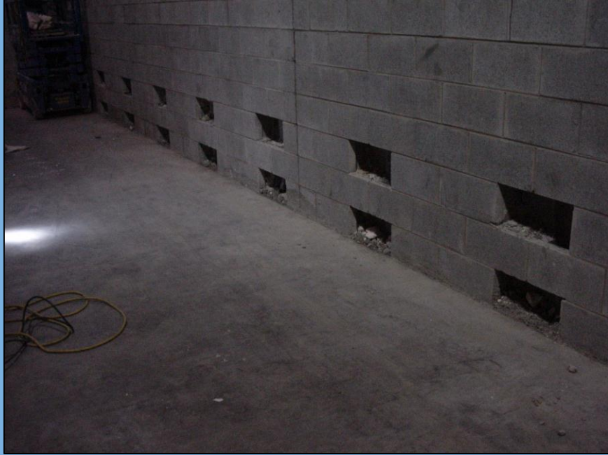
CMU cells removed for base
