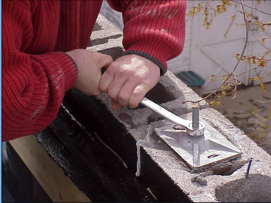
Tensioning rod
