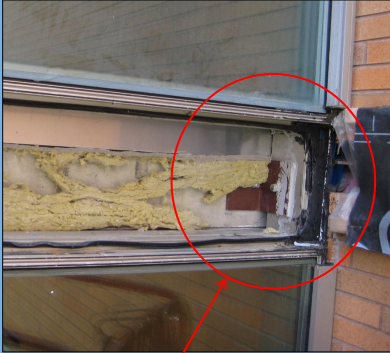
Discontinuity in air barrier
