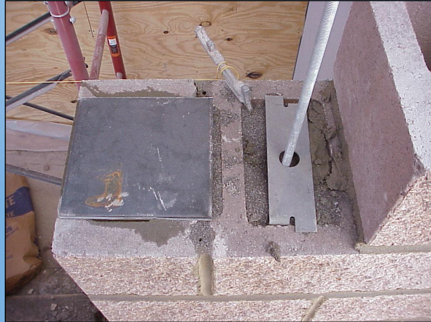
Bar restrainer installation
