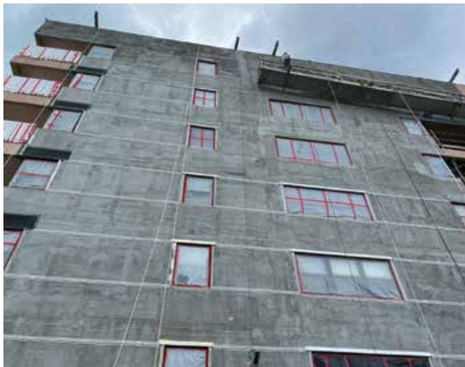
Fig. 8: Stucco installation in progress
