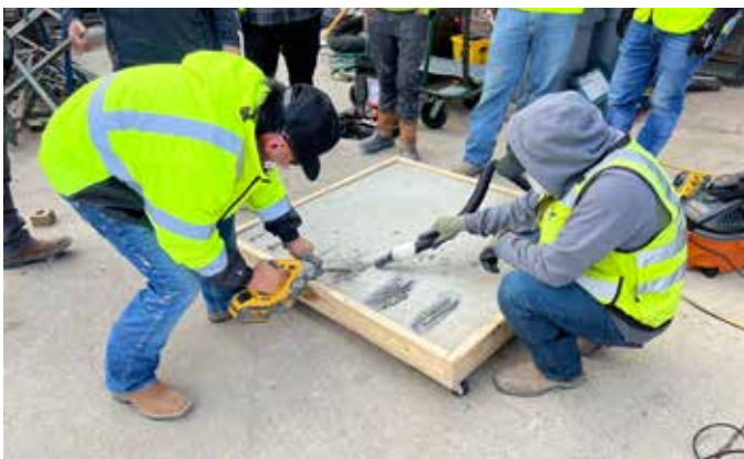
Fig. 4: Removing concrete from around reinforcing bars
