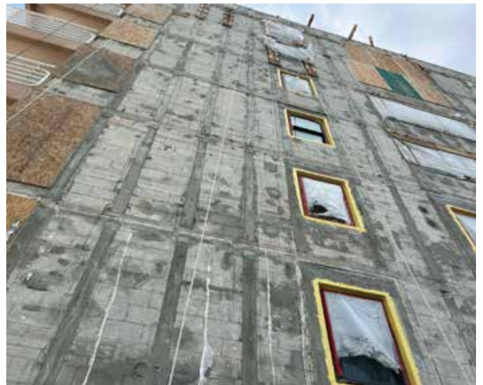
Fig. 7: Completed structural strengthening at the exterior of the building
