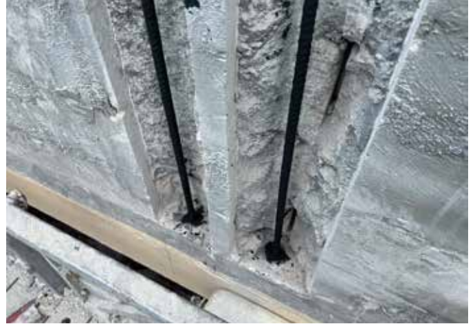
Fig. 6: Structural strengthening installation at the exterior of the building
