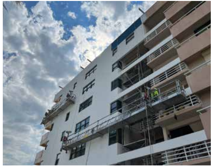
Fig. 9: Elastomeric coating installation in progress
