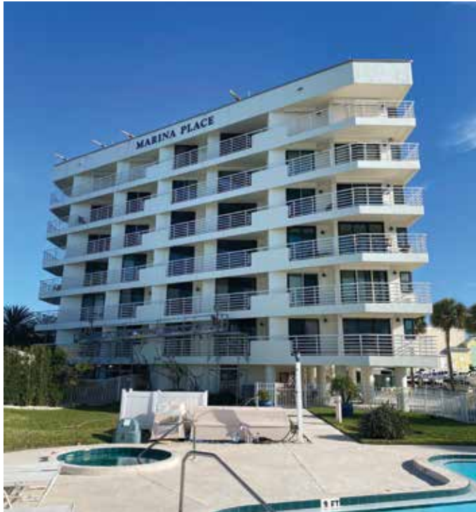
Fig. 1: Completed project after structural strengthening and new stucco and waterproofing system
