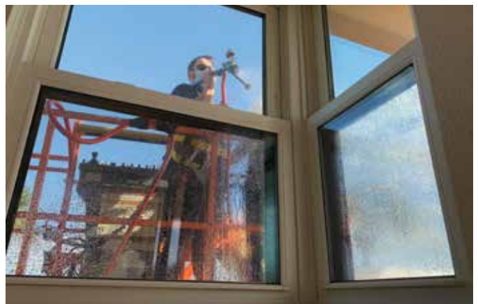
Fig. 3: Water testing at building exterior to replicate Hurricane Eta
