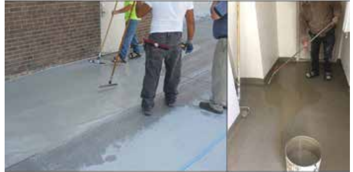
Fig. 7: (a) Cementitious and (b) polyurethane deck coatings
