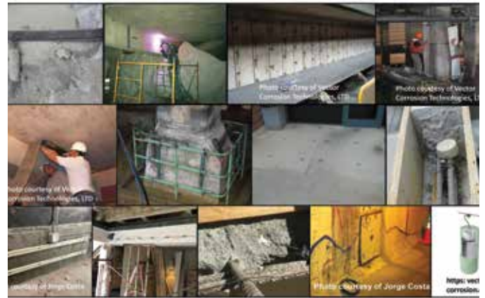
Fig. 9: Cathodic protection systems: (a) MMO-Ti mesh ICCP, (b) thermal spray, (c) discrete anodes, (d) jacketed mesh system, (e) zinc hydrogel sheeting, (f) discrete zinc anodes inside repair, (g) discrete zinc anodes, (h) patch galvanic anode, (i) cassette ICCP system, (j) hybrid ICCP/GCP system with zinc anodes, (k) zinc anodes outside patch area, (l) zinc galvanic panel, and (m) 2-stage ICCP/GCP anode
