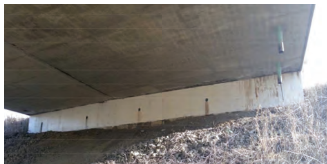
Fig. 10: Abutment of I-75 Bridge over Kirkwood Road (mm 87) in 2022 (Note efflorescence from leaking joint and weep holes)
