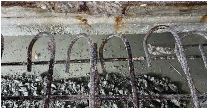
Fig. 5: Cement Paste Remaining on In-Situ Rebar
