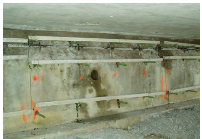
Fig. 5: Dowels and galvanic anodes installed
