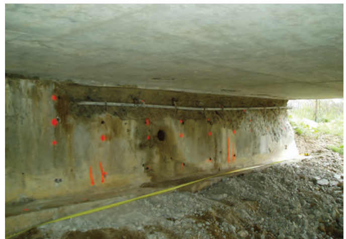
Fig. 4: Concrete spall removal
