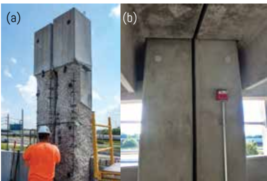
Fig. 8: Column repair (a and b)
