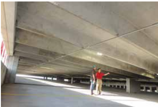
Fig. 7: New double tee beams
