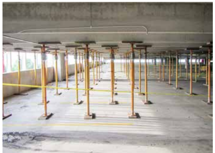
Fig. 4: Shoring installed in affected area
