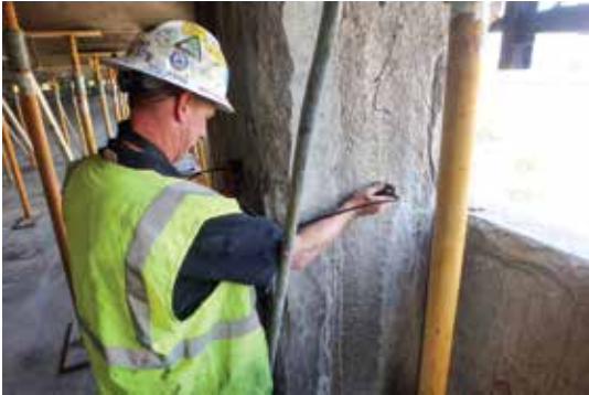
Fig. 5: Nondestructive testing performed at damaged column
