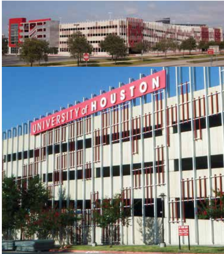
Fig. 1: University of Houston East Garage (top) and fire-damaged area after repair (bottom)
