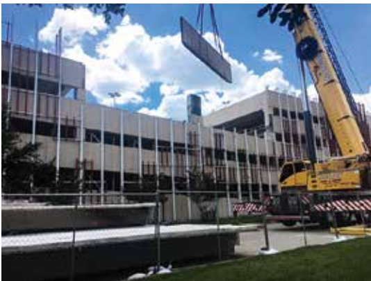
Fig. 6: Spandrel beam replacement
