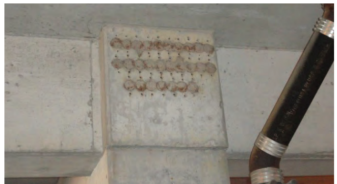
Fig. 5: Corrosion at beam end grout pockets
