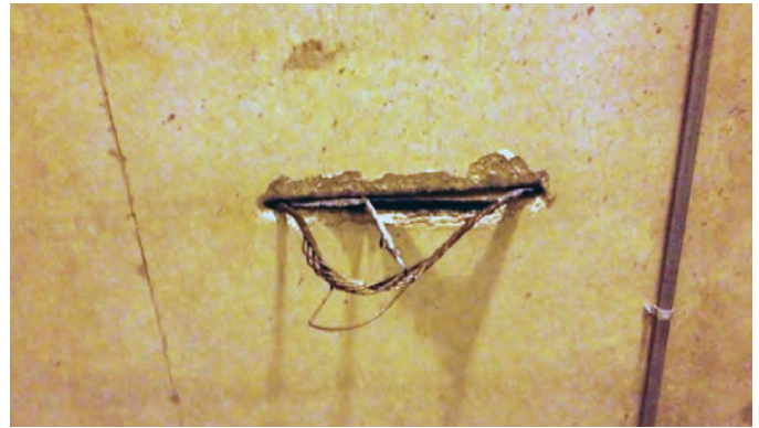
Fig. 2: Erupted post-tensioned tendon discovered March 2013
