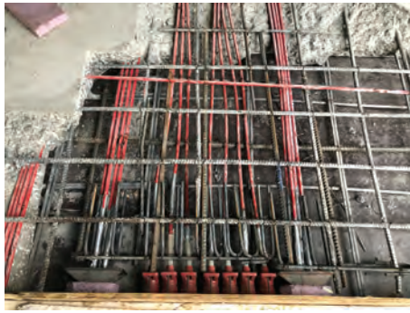
Fig. 7: Modified anchorage detail of banded fifteen (15) tendon bundle at new end anchor location
