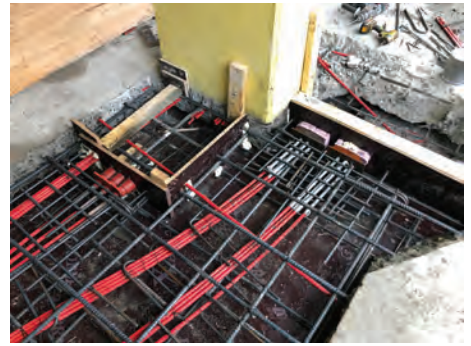
Fig. 8: Modified anchorage detail at column interface
