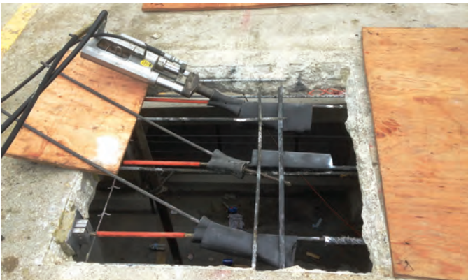
Fig. 8: Post-tension splicing with center stressing chuck
