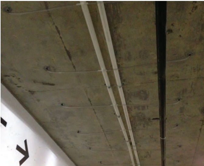
Fig. 11: Manifold system and input air ports for post-tension cable drying
