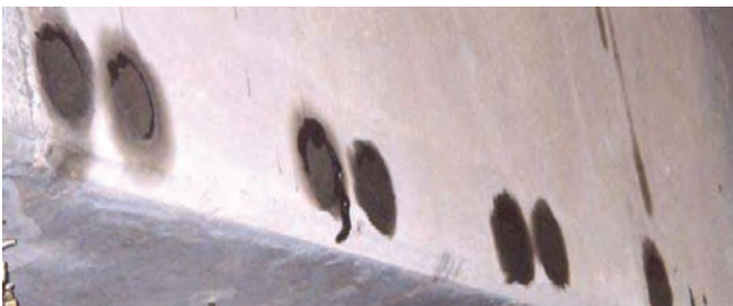
Fig. 14: Post-tension grease at grout pockets
