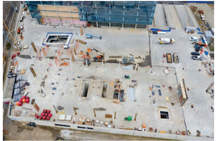
Fig. 2: Gateway Towers 1 and 2 during early construction—PT modification opening shown through the first two levels connecting Tower 1 (already constructed) and Tower 2 (starting concrete frame) (photo courtesy of Baker Concrete Construction)
