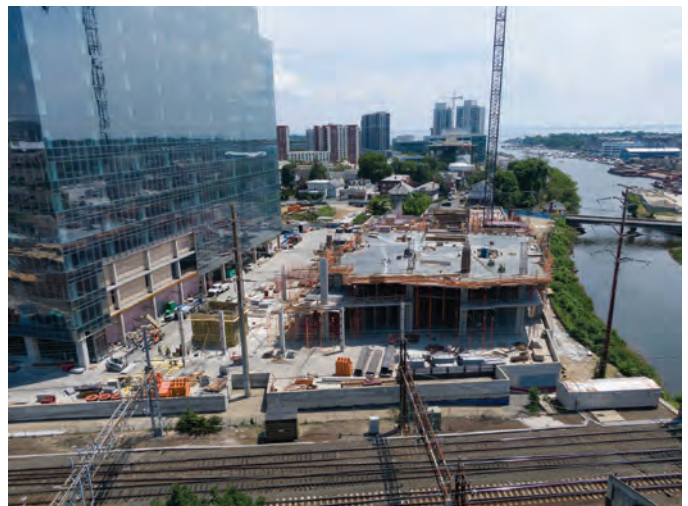
Fig. 3: Gateway Towers 1 and 2 at mid-construction—new core wall construction on the plaza deck between the two new towers (photo courtesy of Baker Concrete Construction)
