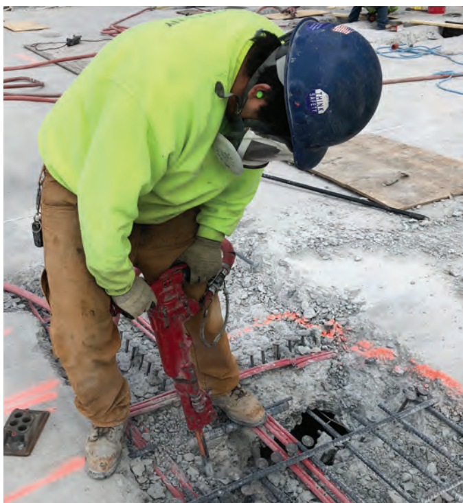
Fig. 5: Removing concrete around existing PT tendons on the Plaza Level
