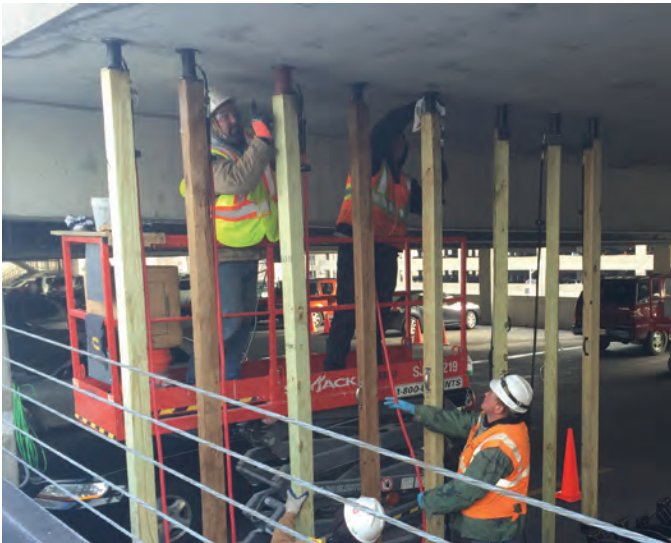
Fig. 13: Post-tension grease injection
