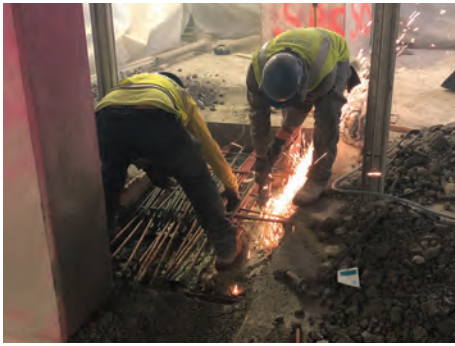
Fig. 6: Controlled de-tensioning of existing PT tendons on Level P2
