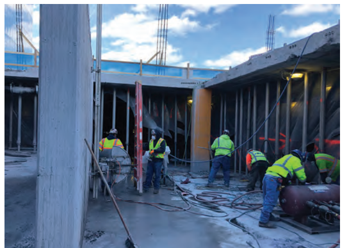
Fig. 4: Shoring, pocket demolition and other PT modifications on Level P1 with the Plaza Level already open above—note number of stressing pockets in the slab
