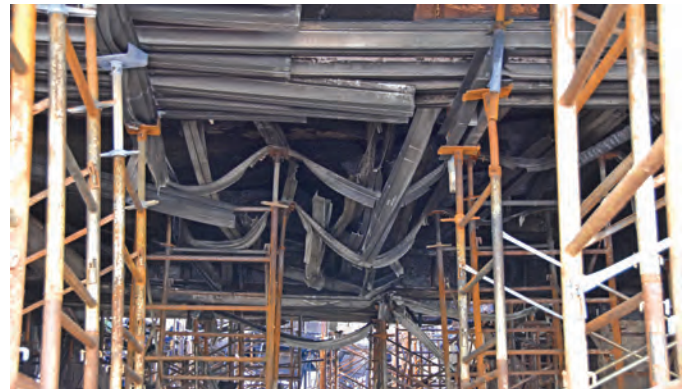
Fig. 4: Melted framework resulting from the intense heat of the flames
