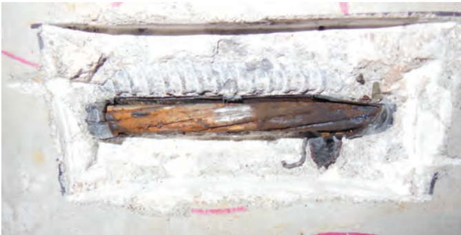
Fig. 7: Severe corrosion and degraded grease
