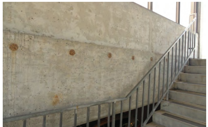
Fig. 4: Corrosion at slab grout pockets
