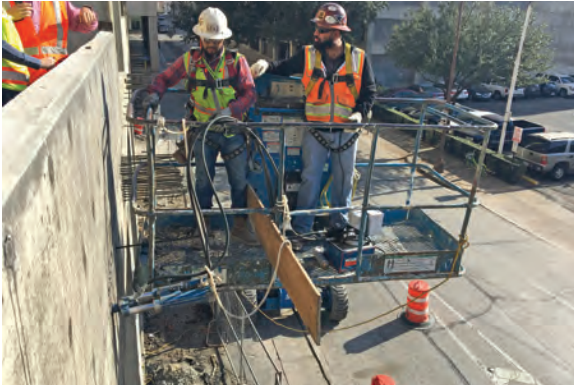
Fig. 7: Initial post-tensioned strand testing
