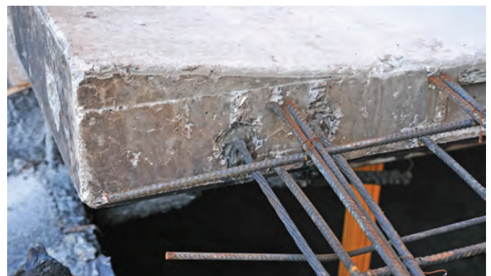
Fig. 6: Ramp slab with melted post-tension encapsulation
