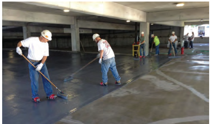
Fig. 10: Application of waterproofing membrane
