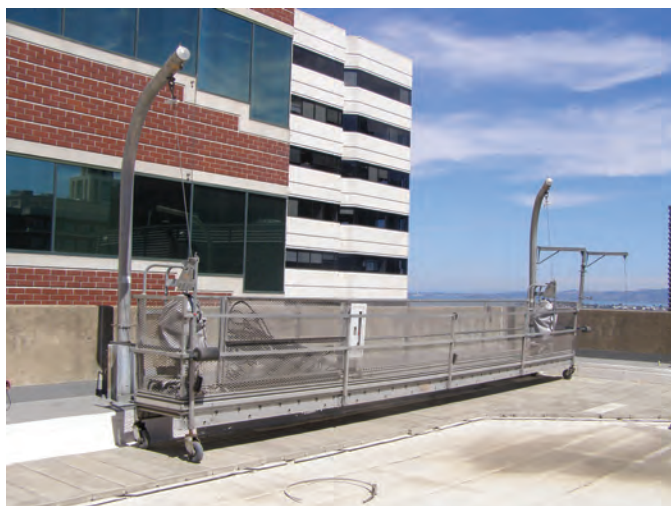
Fig. 2: Davit system and suspended platform (stored on roof)
