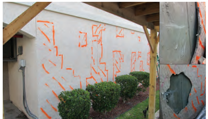
Fig. 4: Debonded stucco identified from audible sounding survey (inset photos at right show subsurface conditions in debonded areas)
