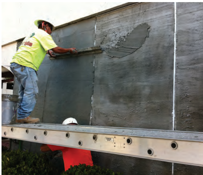
Fig. 11: Application of stucco during repair
