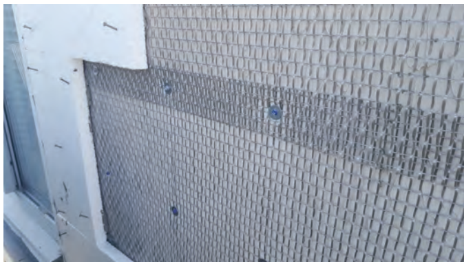
Fig. 13: Existing stucco secured with mesh and anchors for EIFS overcladding (EIFS at left)
