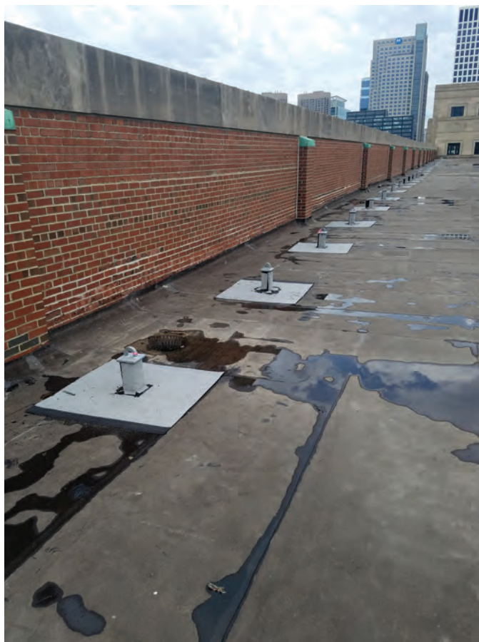
Fig. 3: Dedicated anchorages for securing lifelines
