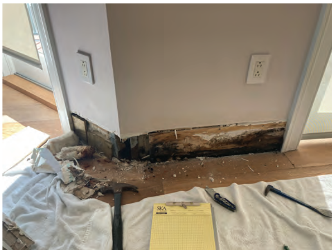
Fig. 6: Interior opening showing significant moisture damage at base of CMU wall
