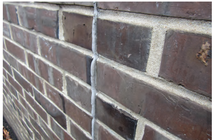
Fig. 7: Sealant pushed out of joint due to thermal movement of brick
