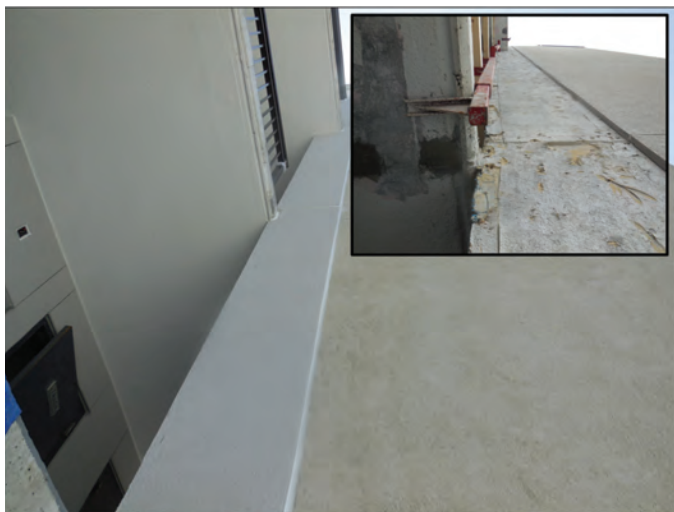
Fig. 12: Repair area showing linear transition and sealants between new and existing stucco (inset shows the extent of the repair area)
