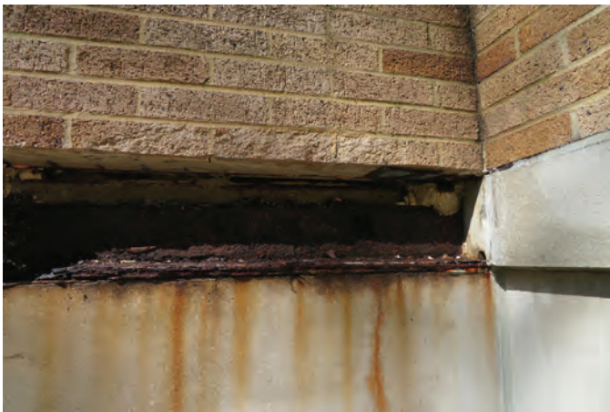
Fig. 4: Corroded shelf angle exposed during exploratory probe
