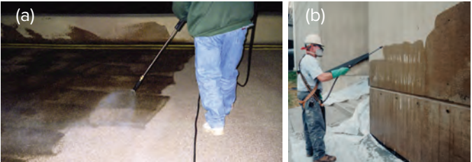
Fig. 2: SAKI spray application to (a) horizontal surface and (b) vertical surface (images courtesy of Sika Corp)
