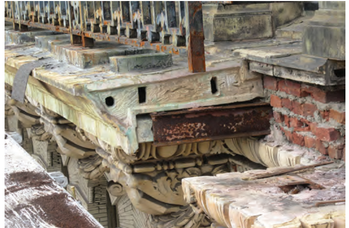
Fig. 6: Terra cotta removed exposing corroded steel support system
