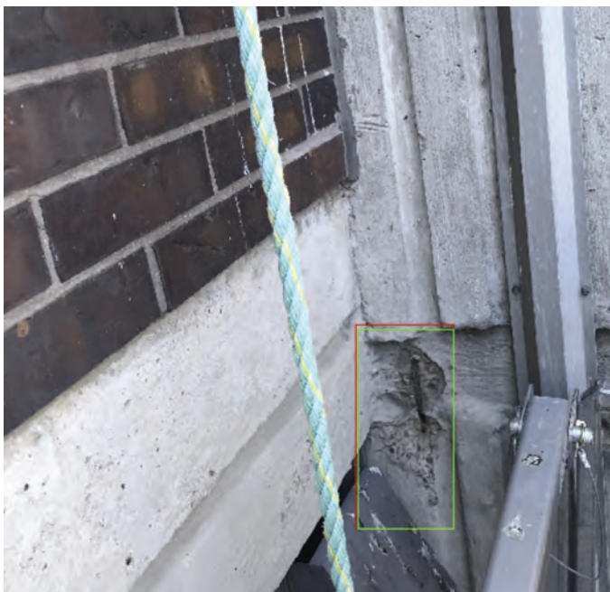
Fig. 4: Double positive indication—spall and exposed rebar
