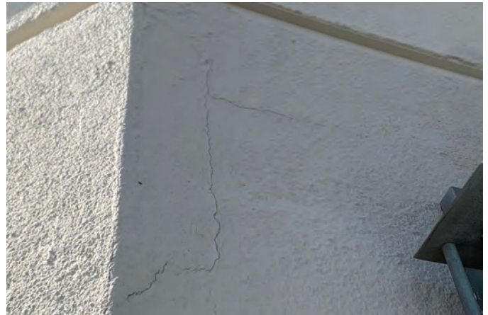
Fig. 3: Cracking in coatings on stucco
