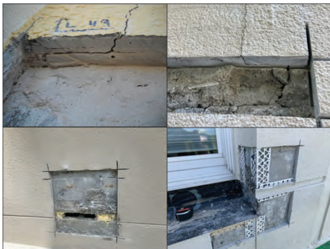
Fig. 7: Exploratory excavations showing cracks through stucco and subparallel to the stucco surface (top), masonry/slab transition with improper spray foam filler (bottom left) and improperly installed window flashing (bottom right)
