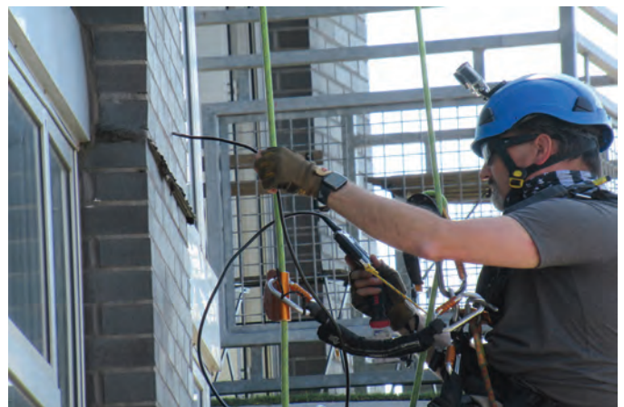
Fig. 8: Inspector using a borescope to view backup construction
