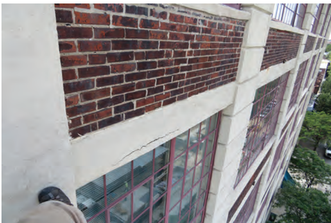
Fig. 5: Delaminated concrete with potential to break free from façade
