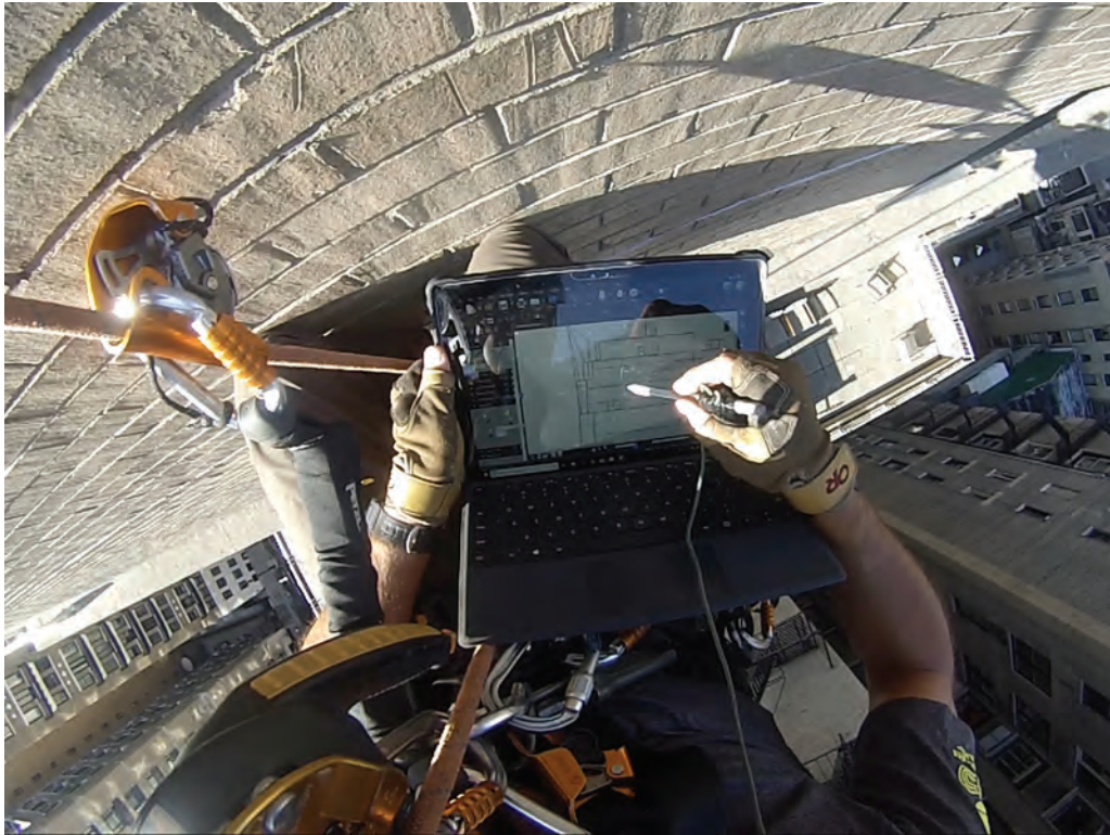
Fig. 1: Engineer performing façade inspection using industrial rope access
