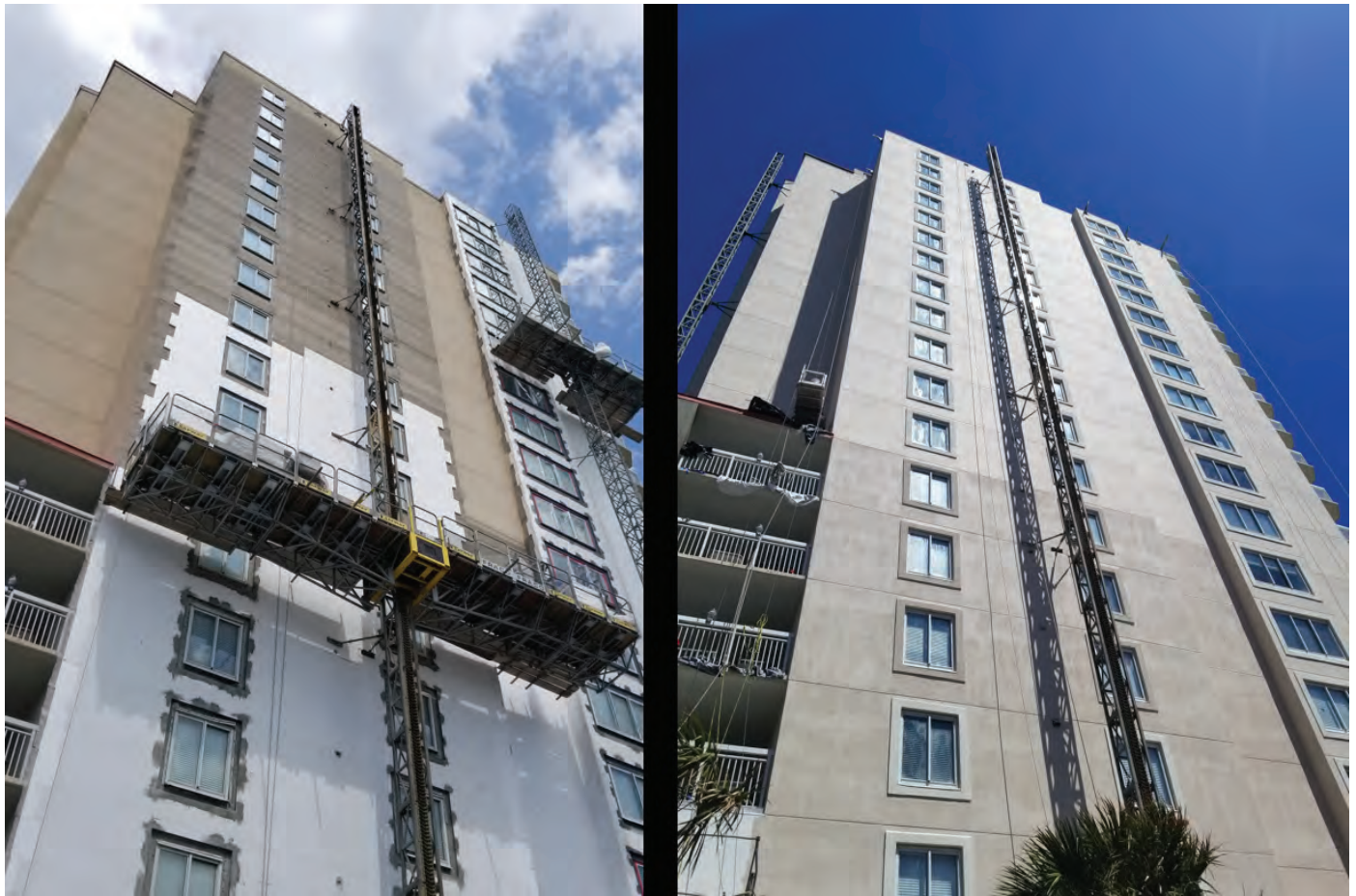
Fig. 14: EIFS being installed over secured stucco (left) and finished wall section with exterior coatings (right)
