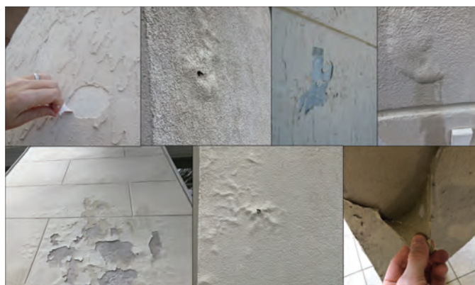
Fig. 9: Coating distress (photo at lower right is an intercoat adhesion failure of coating directly applied to reinforced concrete)
