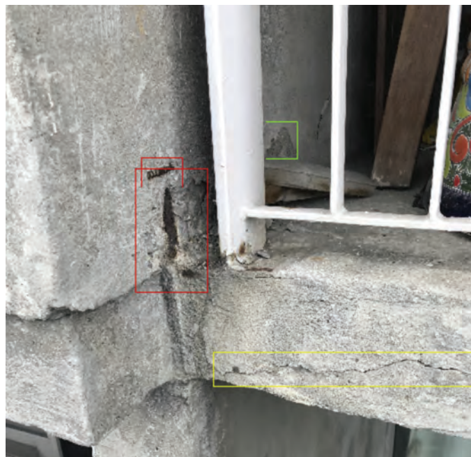
Fig. 5: Example of AI condition detection (red boxes display detected exposed rebar, green—spall, yellow—crack)
