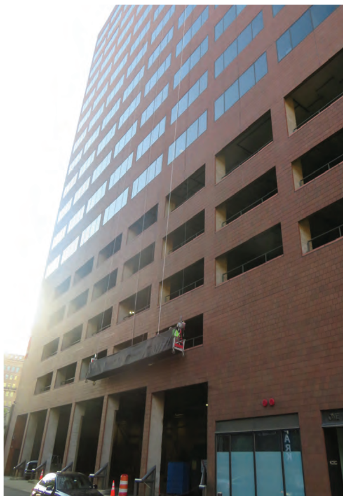
Fig. 3: Swing-stage scaffold erected for façade inspection
