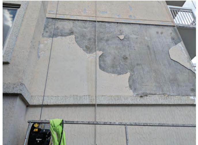
Fig. 2: Debonded stucco on concrete substrate
