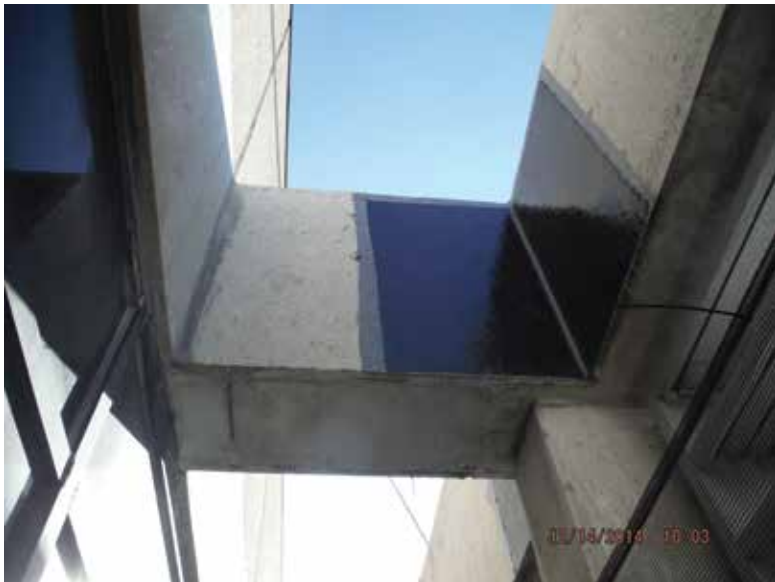
Fig. 7: CFRP repairs on sunshade beam flange and web
