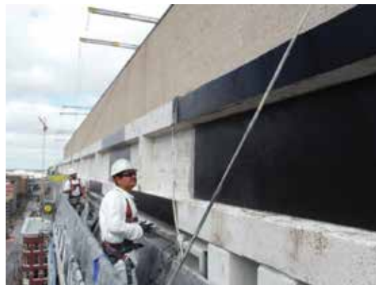
Fig. 5: Swing stage equipment used for CFRP repairs
