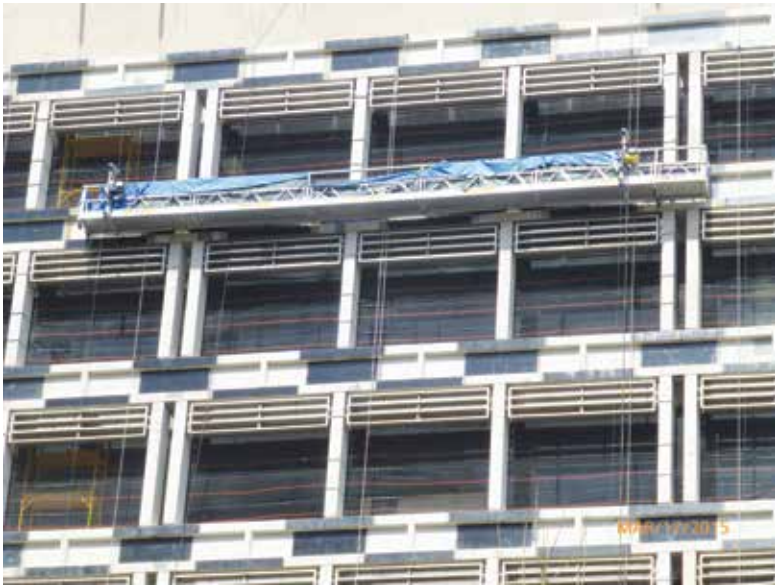
Fig. 6: CFRP fabric installation at exterior web faces
